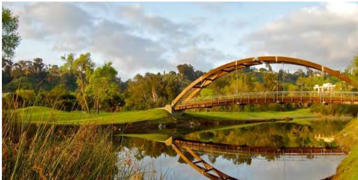
Existing bridge across the San Diego River
