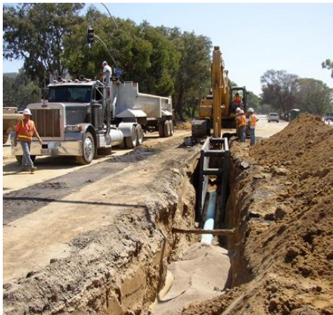
Trenching the municipal sewer
