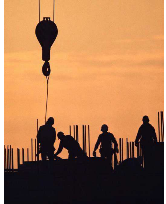
Capital improvements under construction
