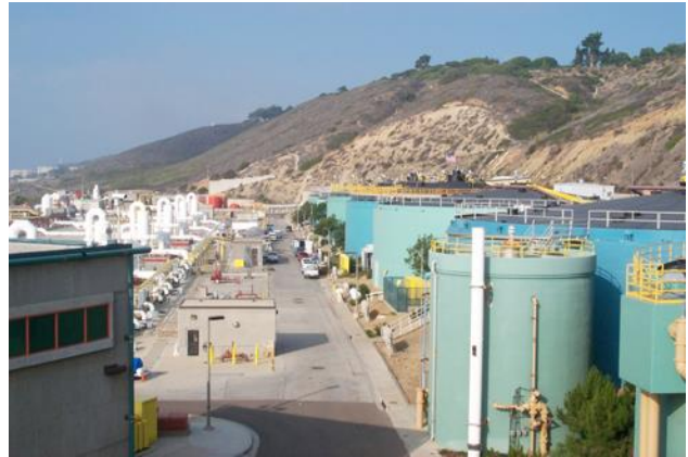
Point Loma Wastewater Treatment Plant
