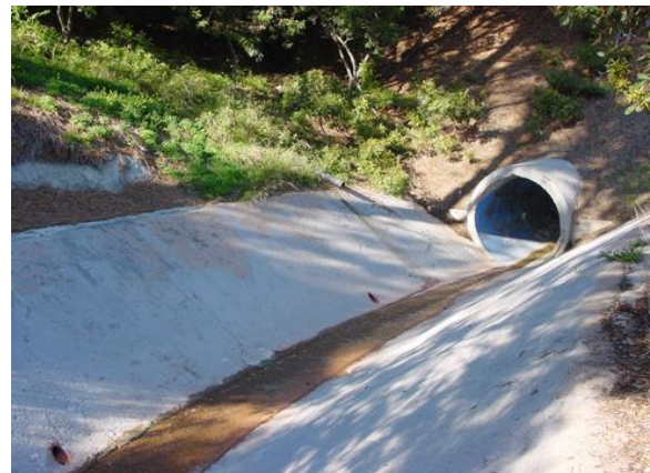
City of San Diego storm drain
