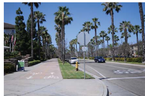
Example of a raised cycle-track
