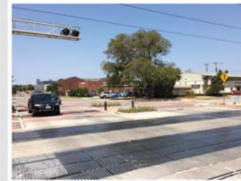
Train crossing is clearly demarcated as a separate area from pedestrian crosswalk
