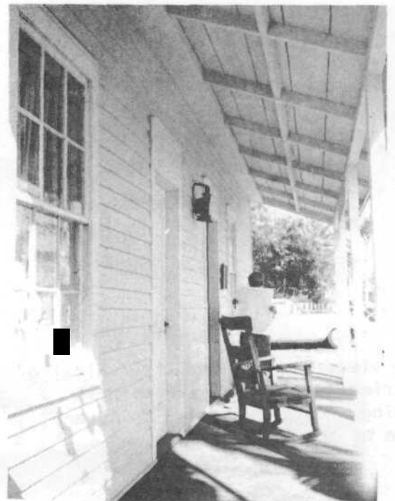
Close-up view of 1yp double-hung window, door and wall siding.
