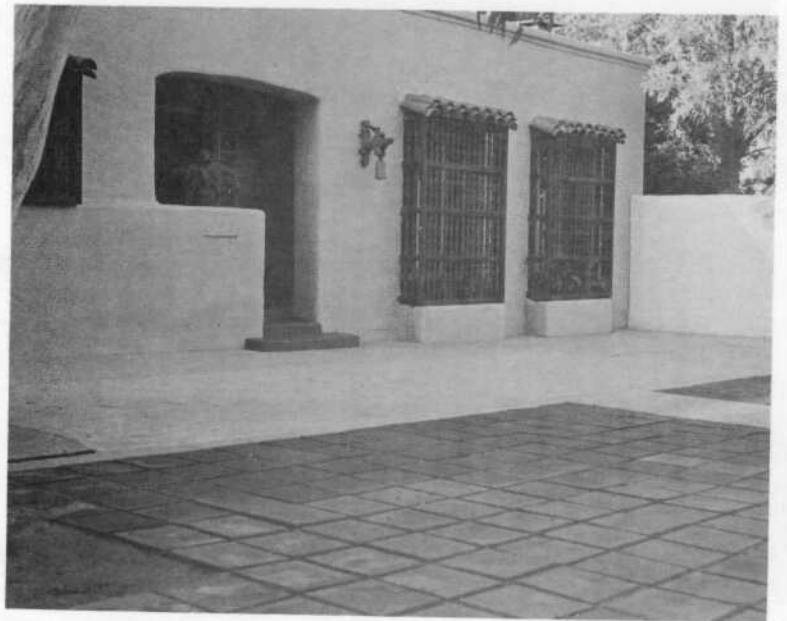
Varied street treatment. Characteristic coping treatment without tile roof decoration or overhang, yet is very effective. Tile treatment above window. Spool design wood grille over window is typical of Spanish influence. Note pleasing effect of shadows over 12" paving tiles of type used during Spanish-Mexican period.
