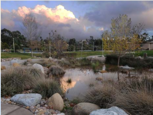
Water Quality Basins capture contaminated Stormwater
