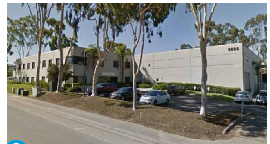
2 Office building located at 9600 Kearny Villa Road, 0.45 FAR.
