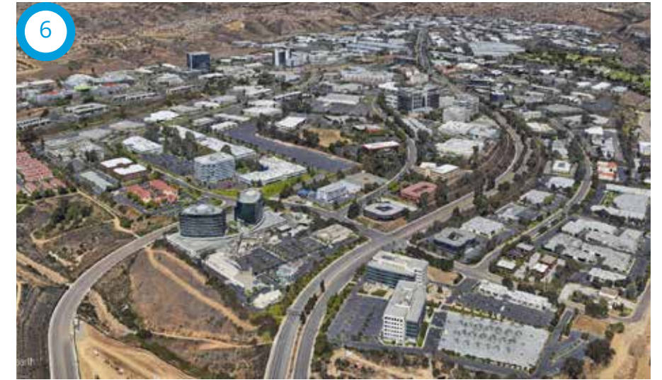
Sorrento Mesa Office/R&D Area
