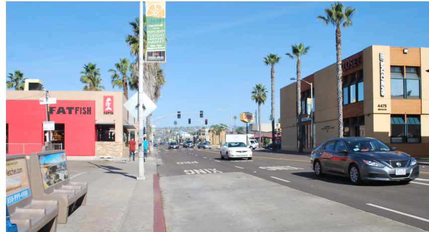
Mission Boulevard and the rest of the study area have a mix of visitor-serving commercial uses, restaurants, retail, hotels, entertainment, and recreation.
