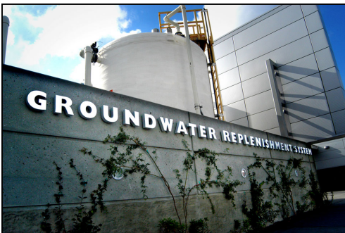
Orange County's water purification facility
