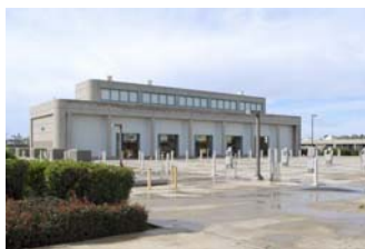
North City Water Reclamation Plant
