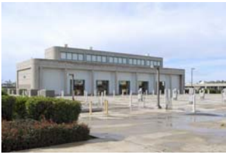
North City Water Reclamation Plant
