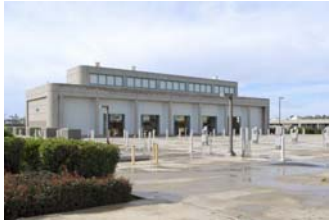
North City Water Reclamation Plant
