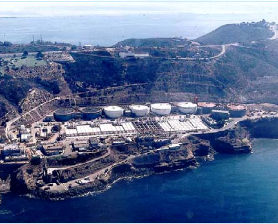
Point Loma Wastewater Treatment Plant
