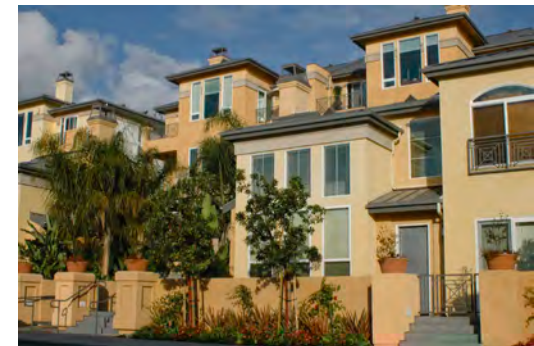
Step back upper stories of a building to diminish the appearance of height on the street.
