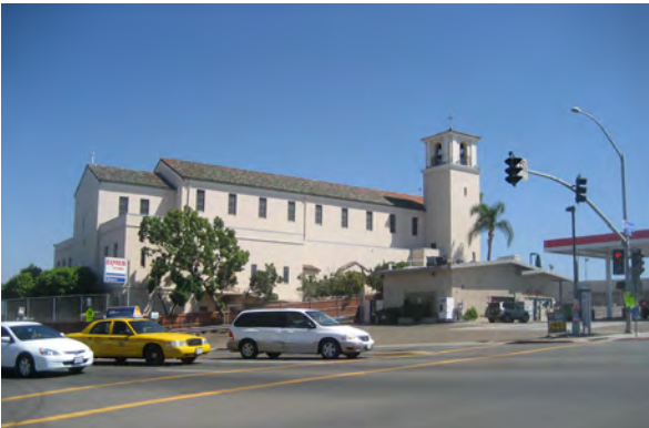
Several iconic buildings contribute to the area's identity and provide a sense of entry into the community.
