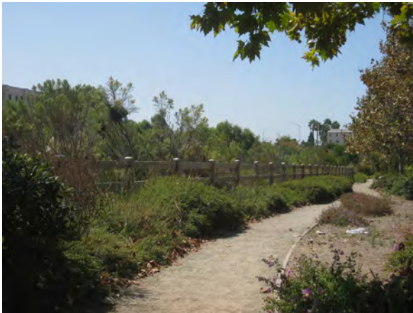
Existing multi-use paths through Valencia Business Park
