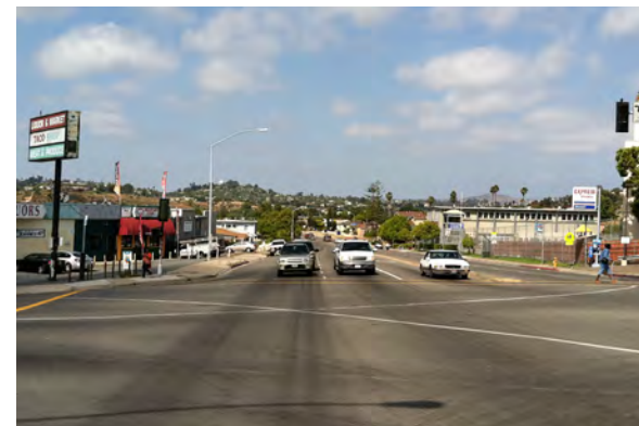
The widths of intersections like Euclid and Imperial are overly wide for pedestrian comfort and safety.
