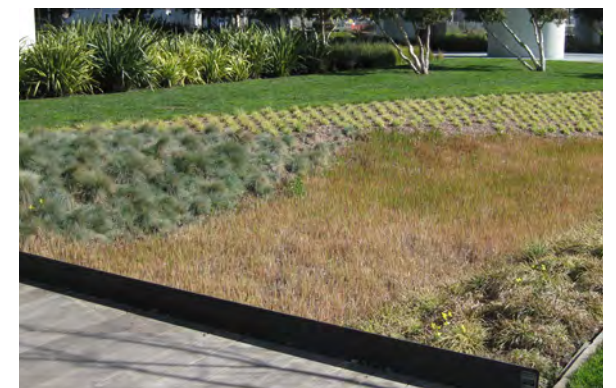
Stormwater Management Feature
