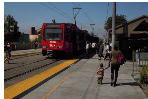
The Euclid and 47th Street Intermodal Transit Stations provide excellent regional access.
