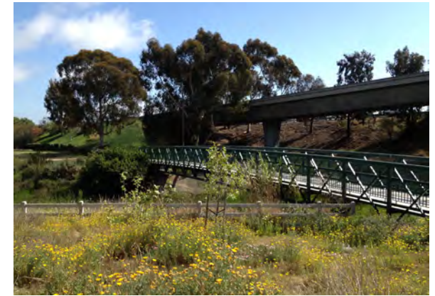
An example of natural park setting with pedestrian bridge.
