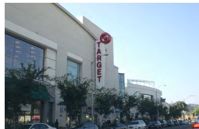
An example of a two-story Target Store that addresses the street and public realm.
