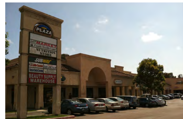
Major retail uses are generally located along Euclid Avenue near Market Street.
