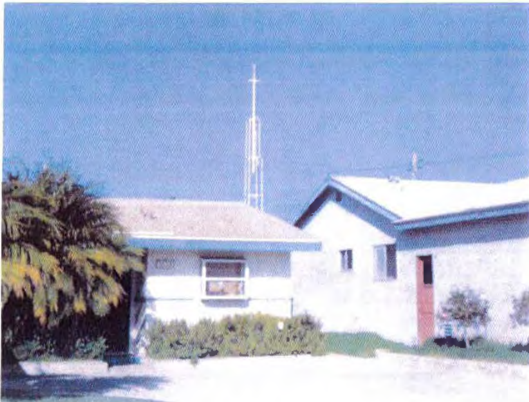
LOOKING NORTHWEST AT SUBJECT TOWER
