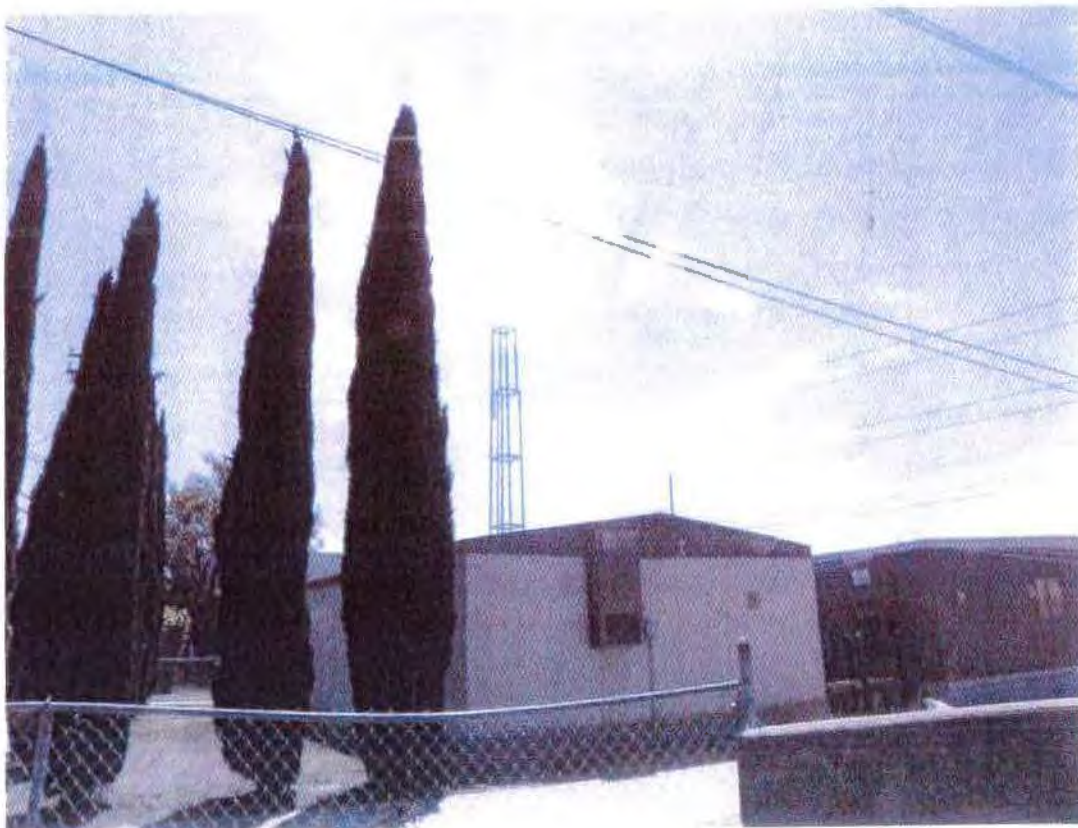
LOOKING SOUTHWEST AT SUBJECT TOWER
