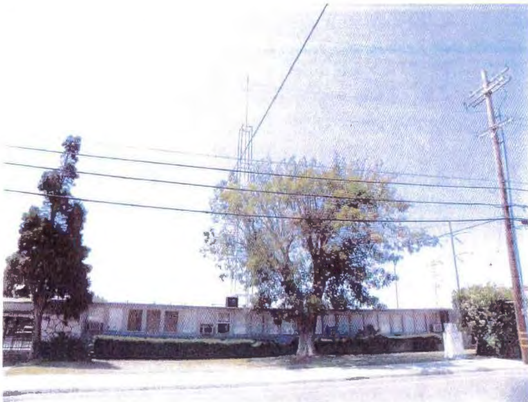
LOOKING WEST AT SUBJECT TOWER
