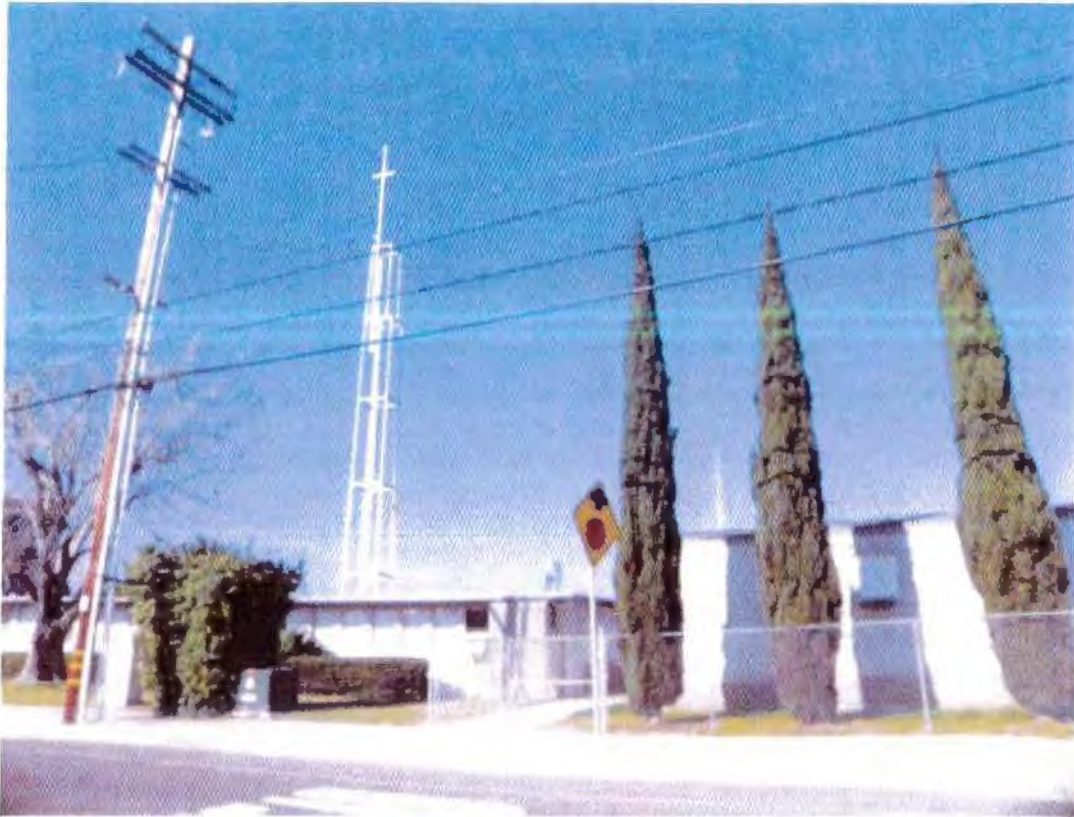
LOOKING SOUTHWEST AT SUBJECT TOWER
