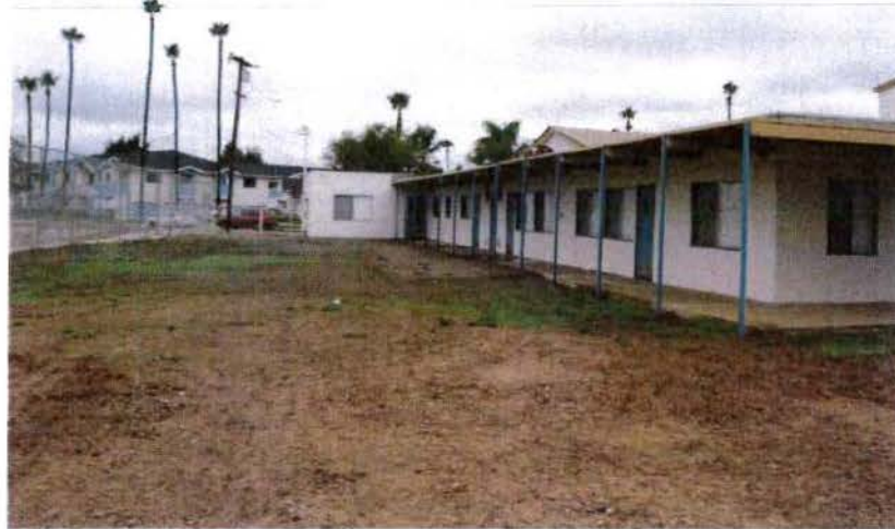
Looking north from site
