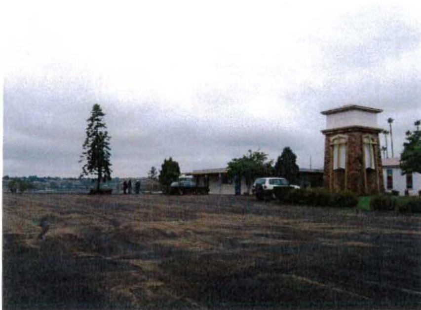
Looking at south elevation
