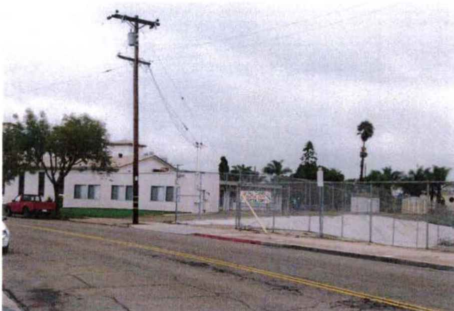
Looking at west elevation
