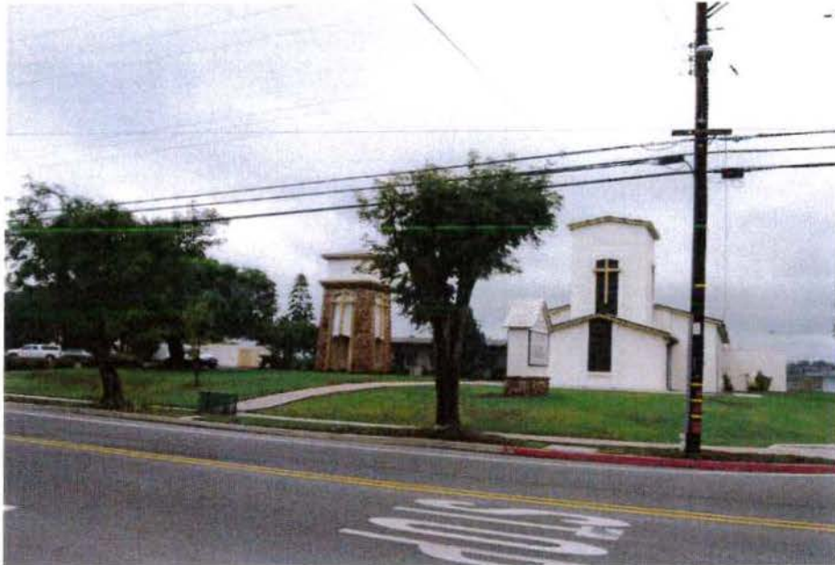
Looking at east elevation
