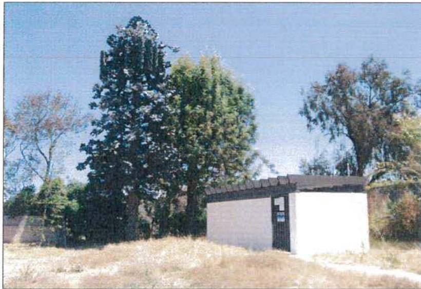
South Elevation (T-Mobile)
