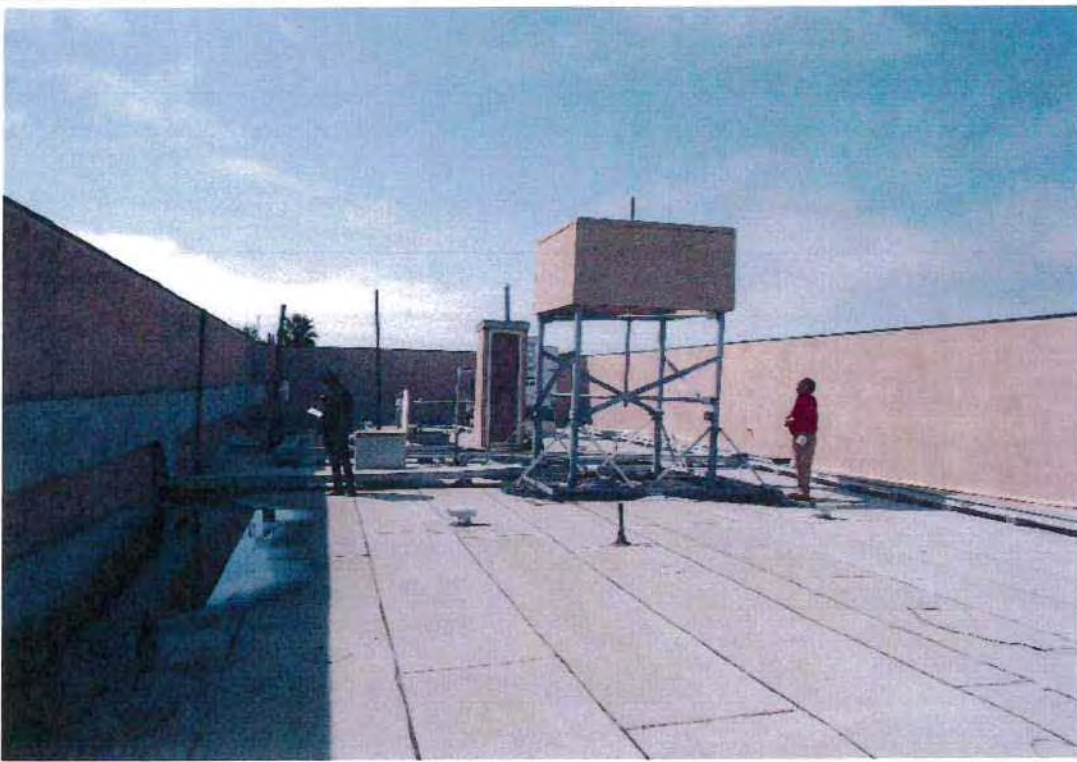
Looking west through roof area
