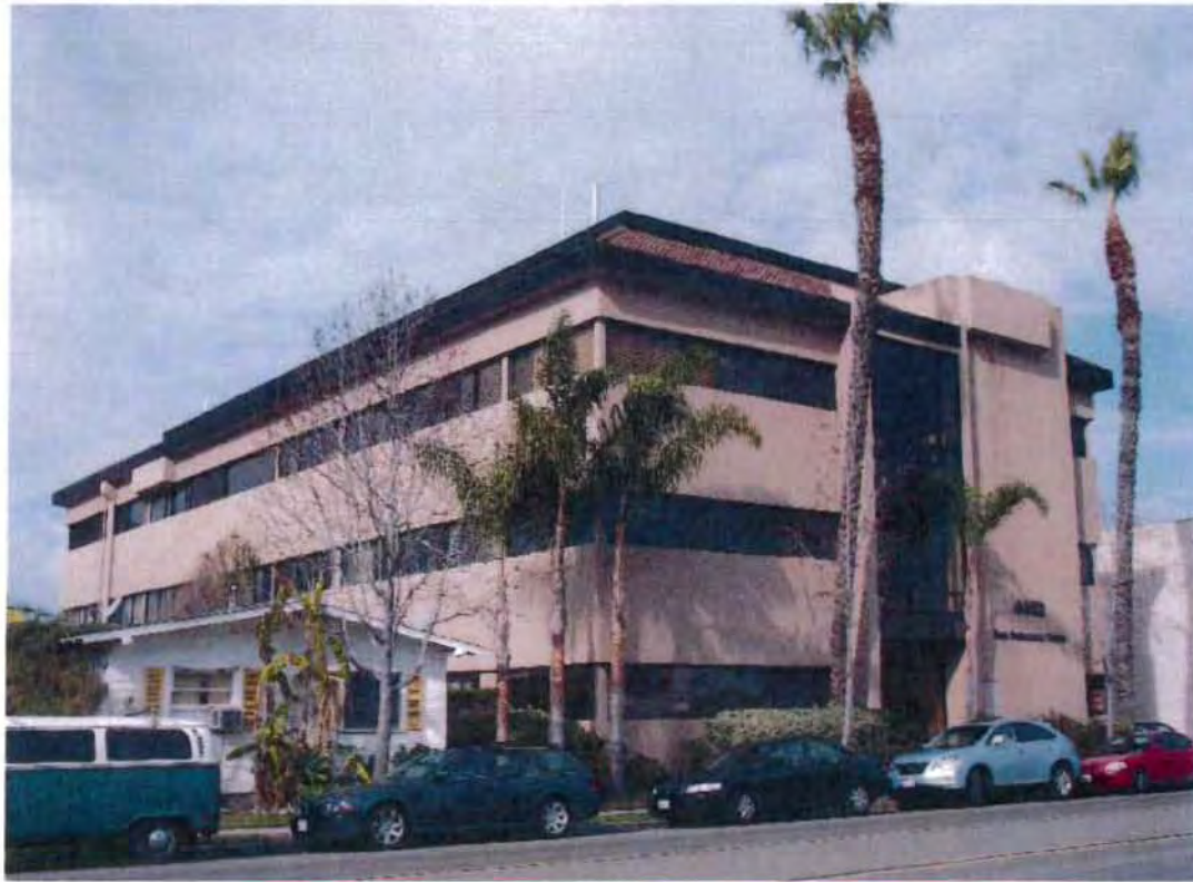
Looking west towards project site
