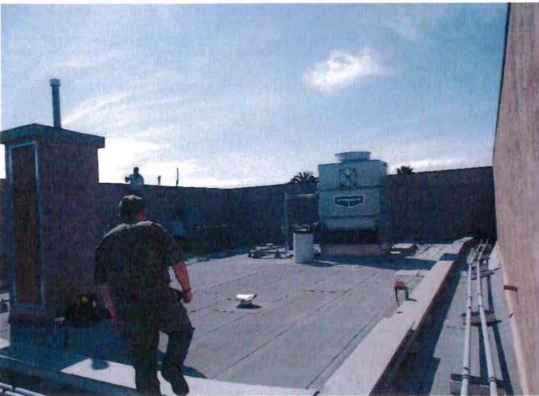
Looking east through roof area
