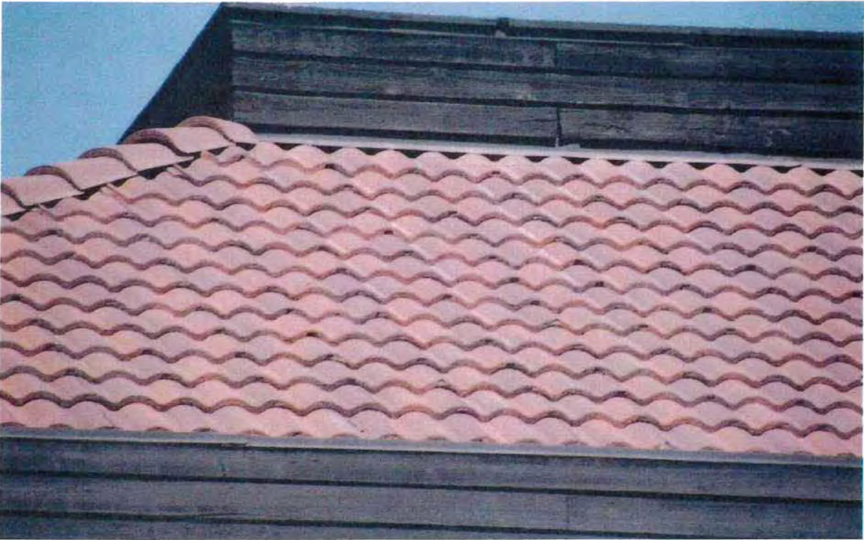
Close up of existing roof parapet
