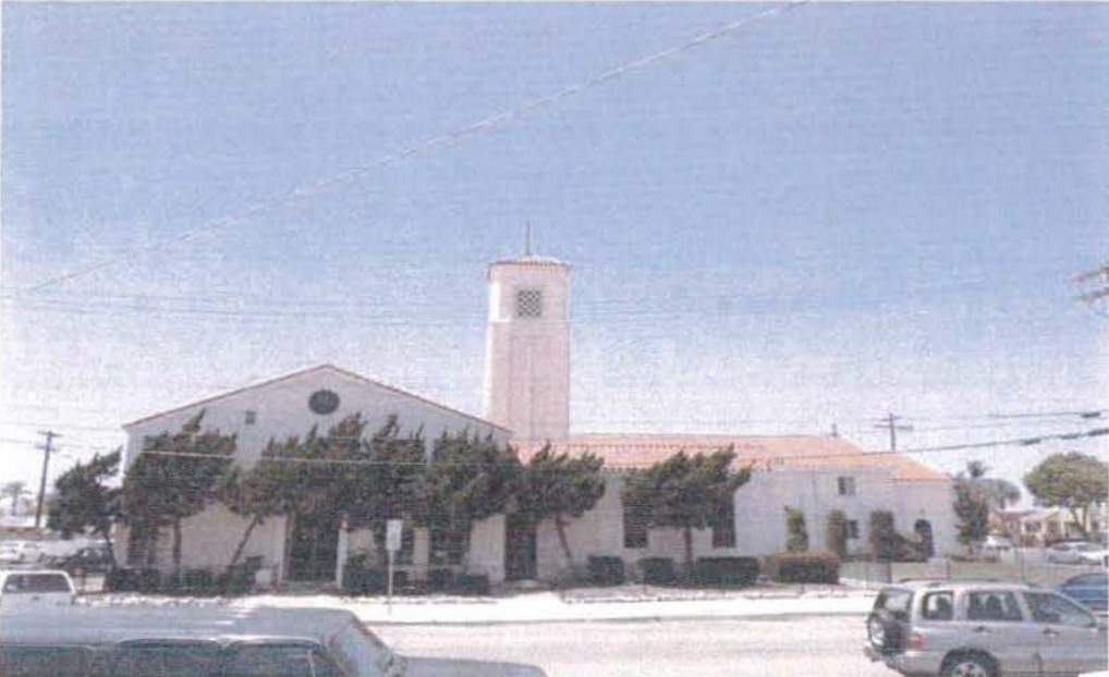
(2) View of the subject property looking west
