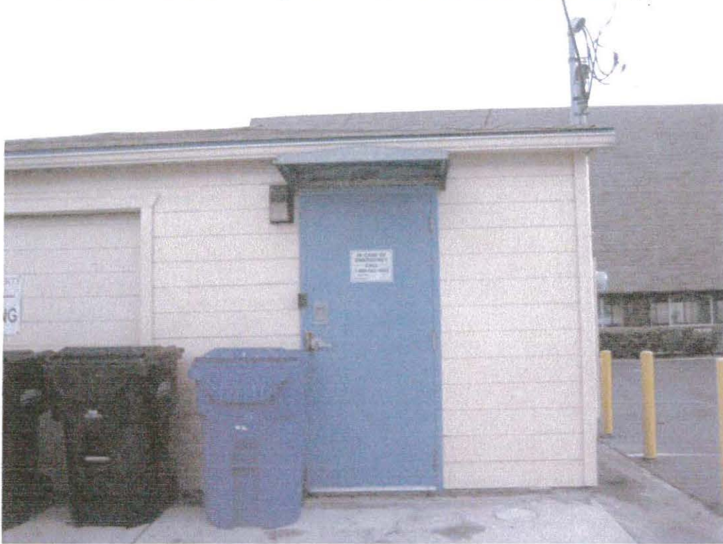
9. View of the exterior of the existing equipment enclosure.
