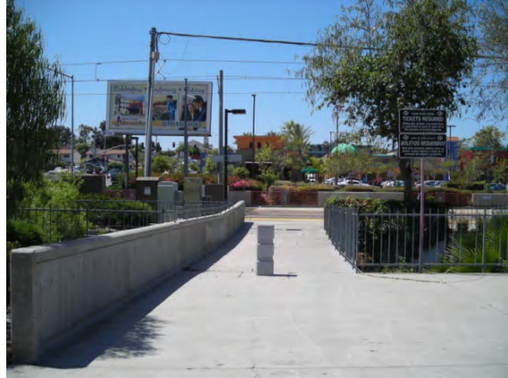
Pedestrian Bridge across Chollas Creek into the Trolley Station
