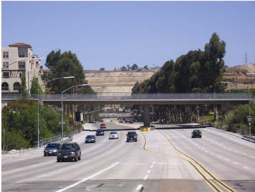
View before project.
