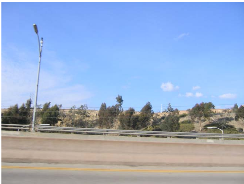
Looking north from Friars Road bridge over Qualcomm Way.
