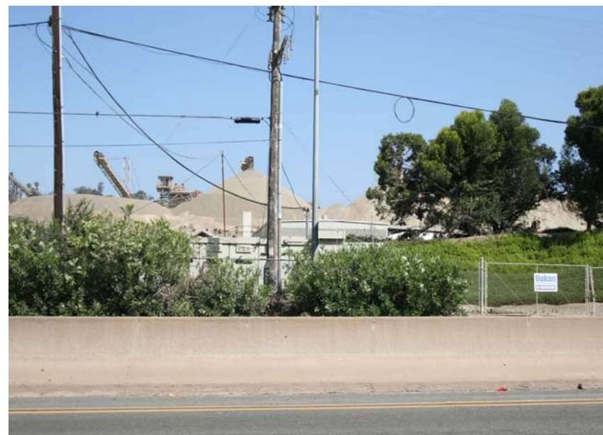
Looking north at west mid portion of site.
