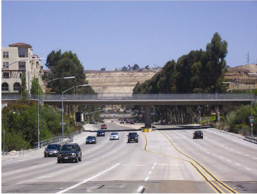
View before project.
