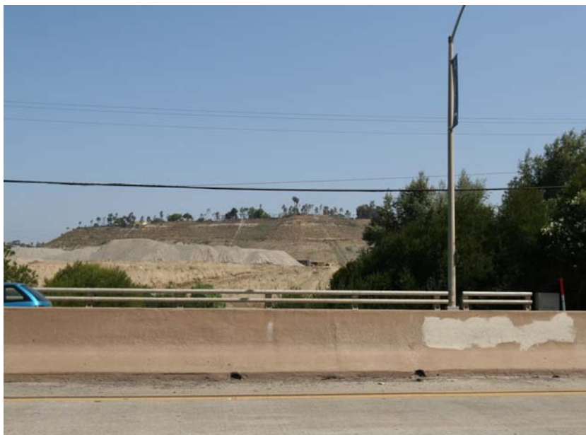
Looking north at west end of project site.
