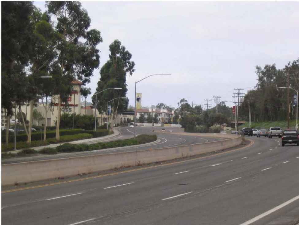
View before project.
