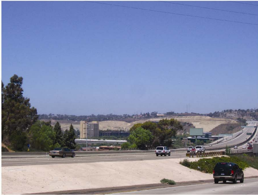
View before project.
