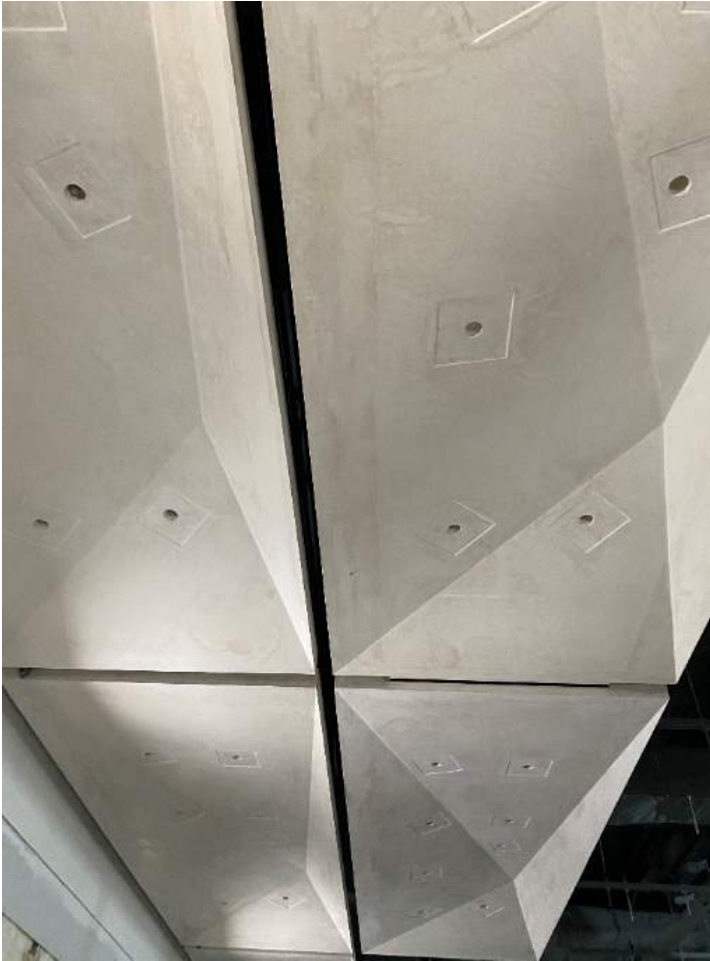
Gallery level custom GFRG ceiling panel progress on the Gallery level along with ongoing framing and MEP rough-in the back ground.
