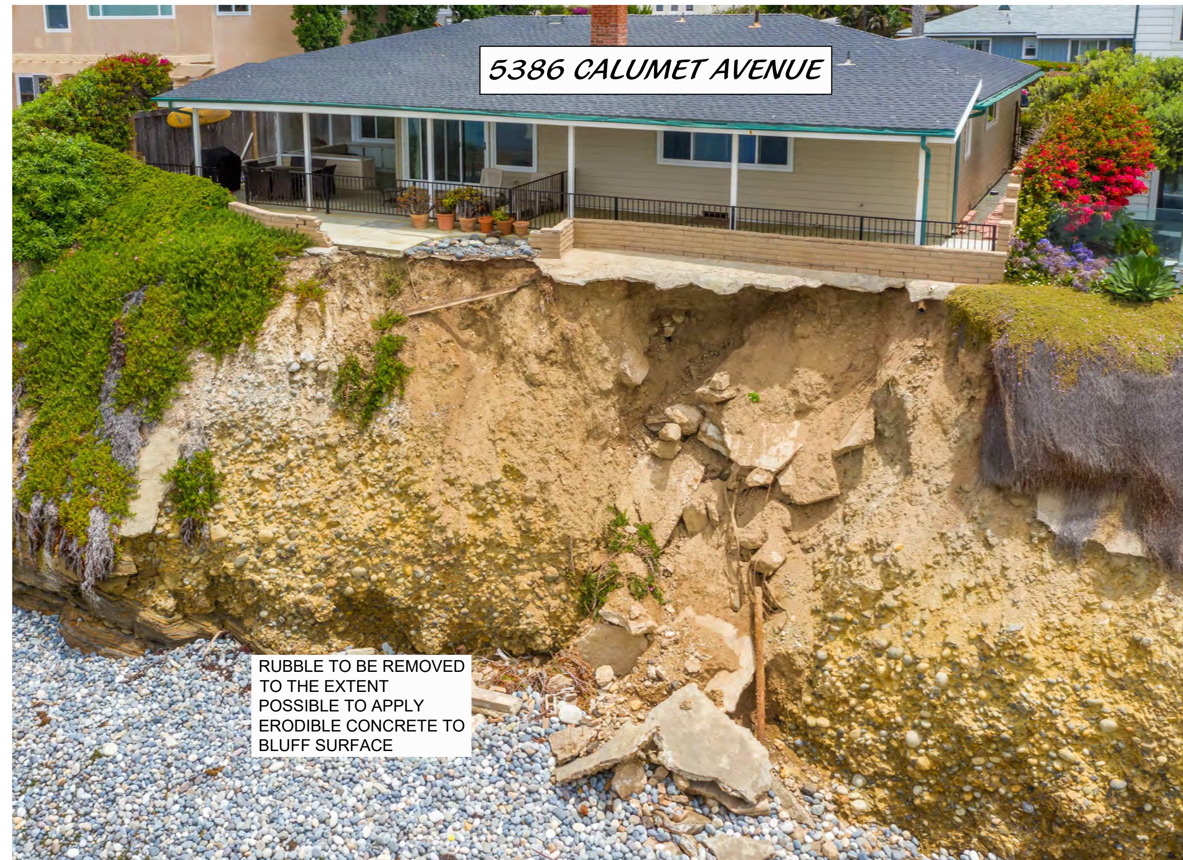
DRONE PHOTO - EXISTING CONDITION
