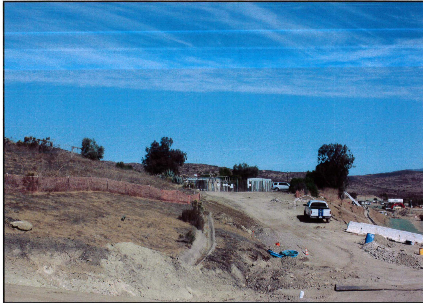
SITE PRIOR TO INSTALLATION
