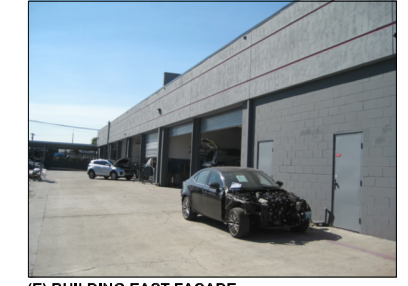
(E) BUILDING EAST FACADE
