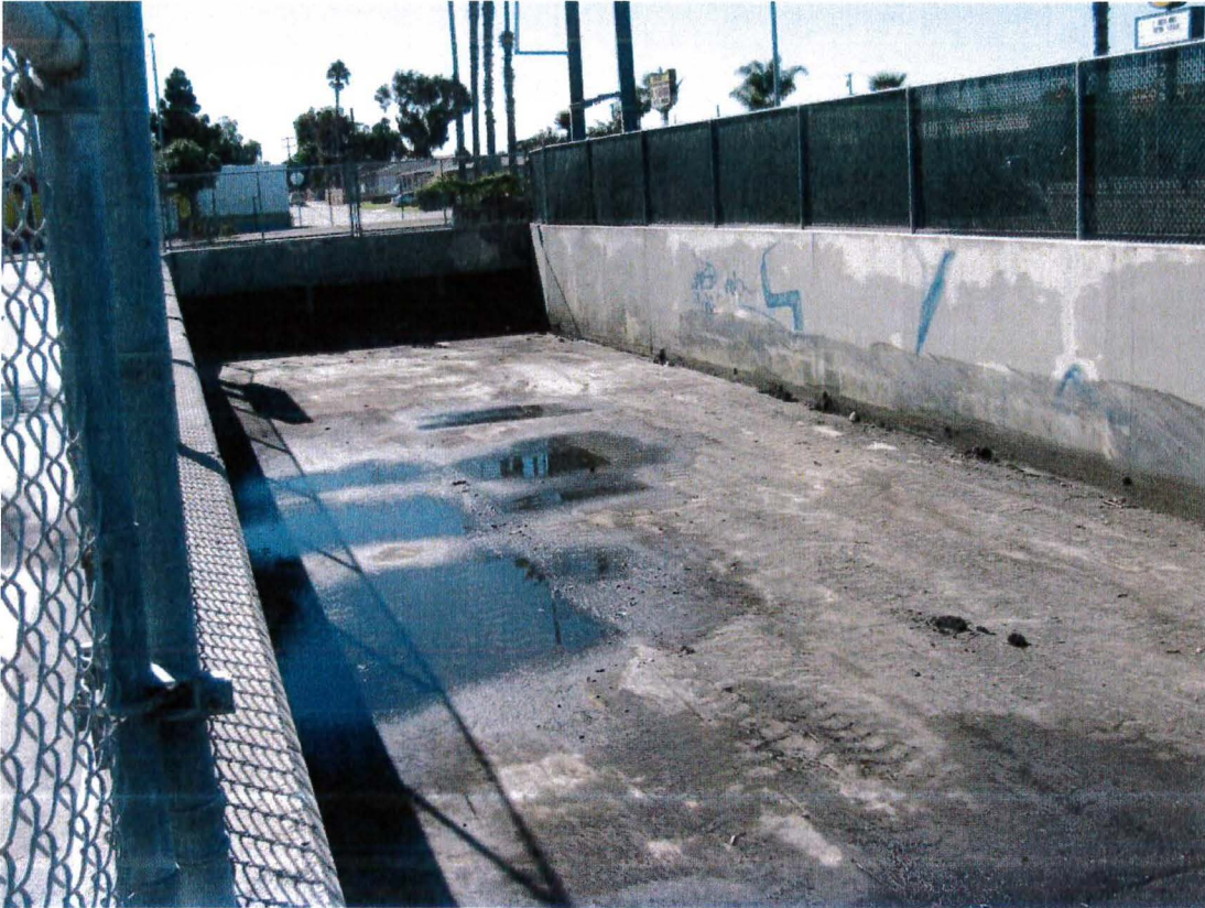
Near upstream end of Nestor Map 134, looking upstream. November 12, 2010
