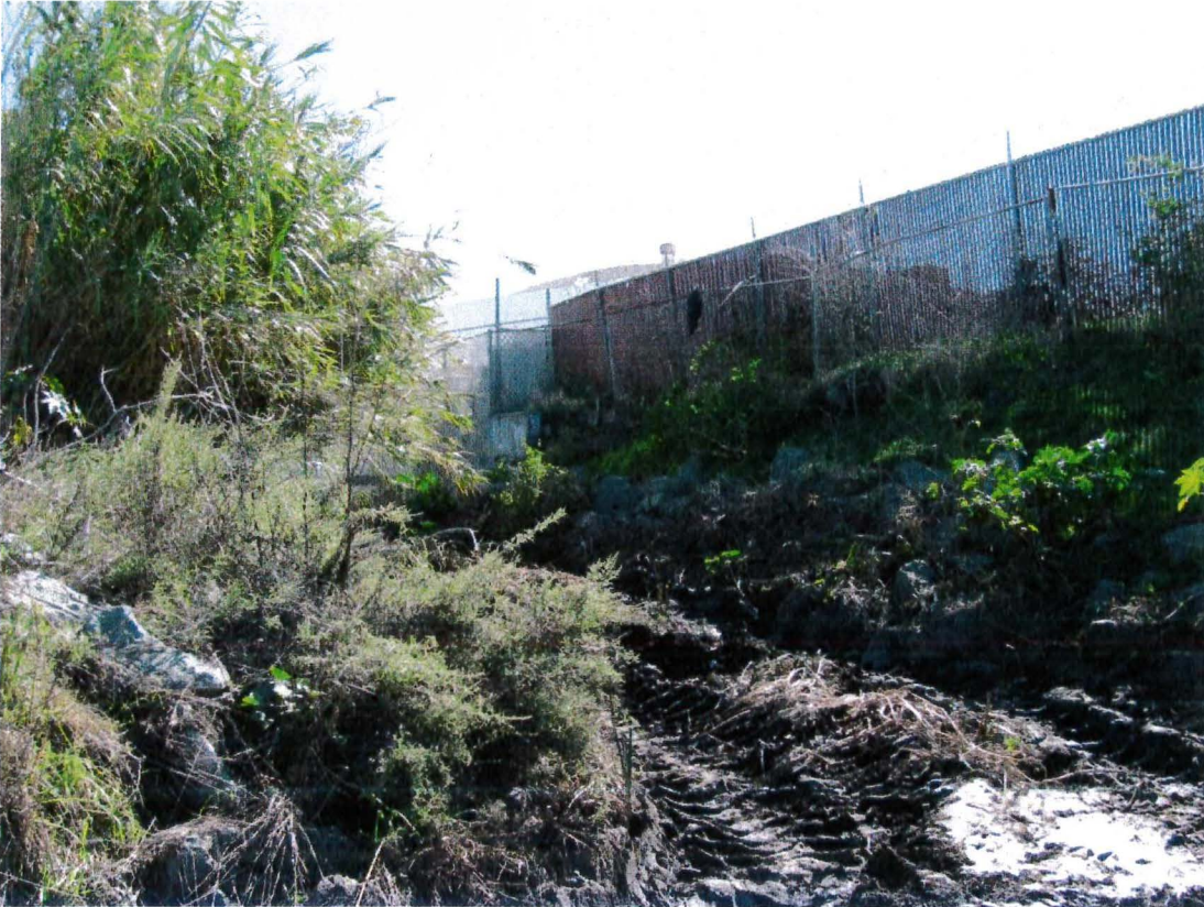
At downstream end of Nestor Map 134 looking upstream. November 12, 2010
