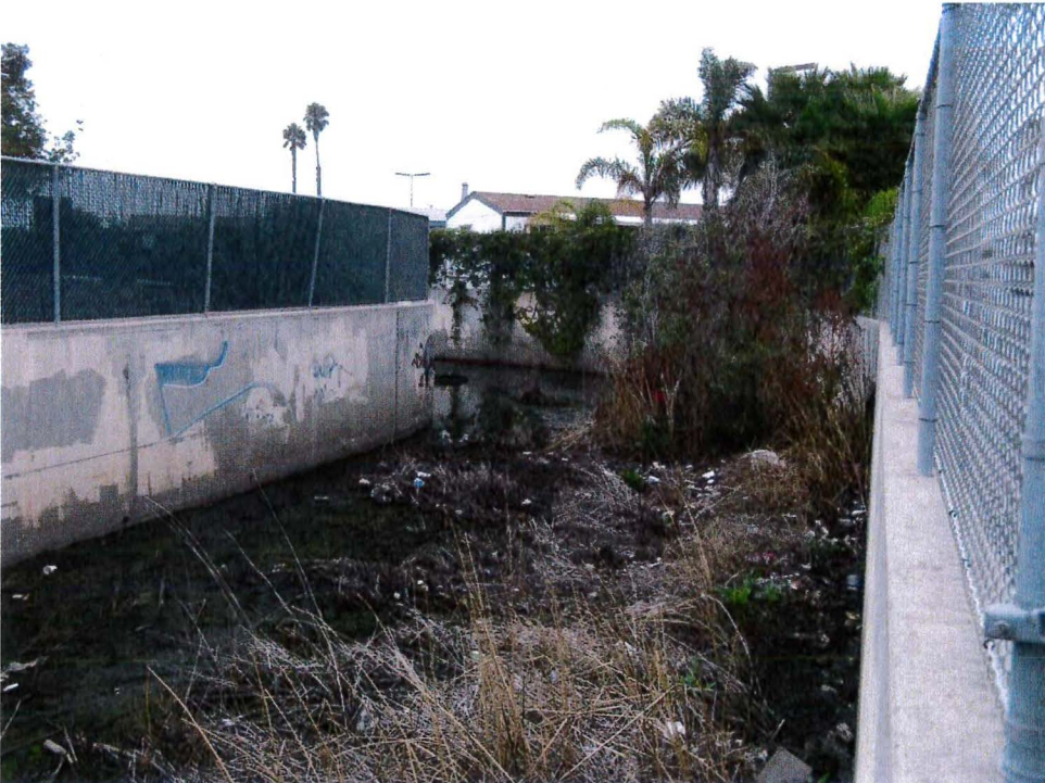
Near upstream end of Nestor Map 134 looking downstream. October 18, 2010
