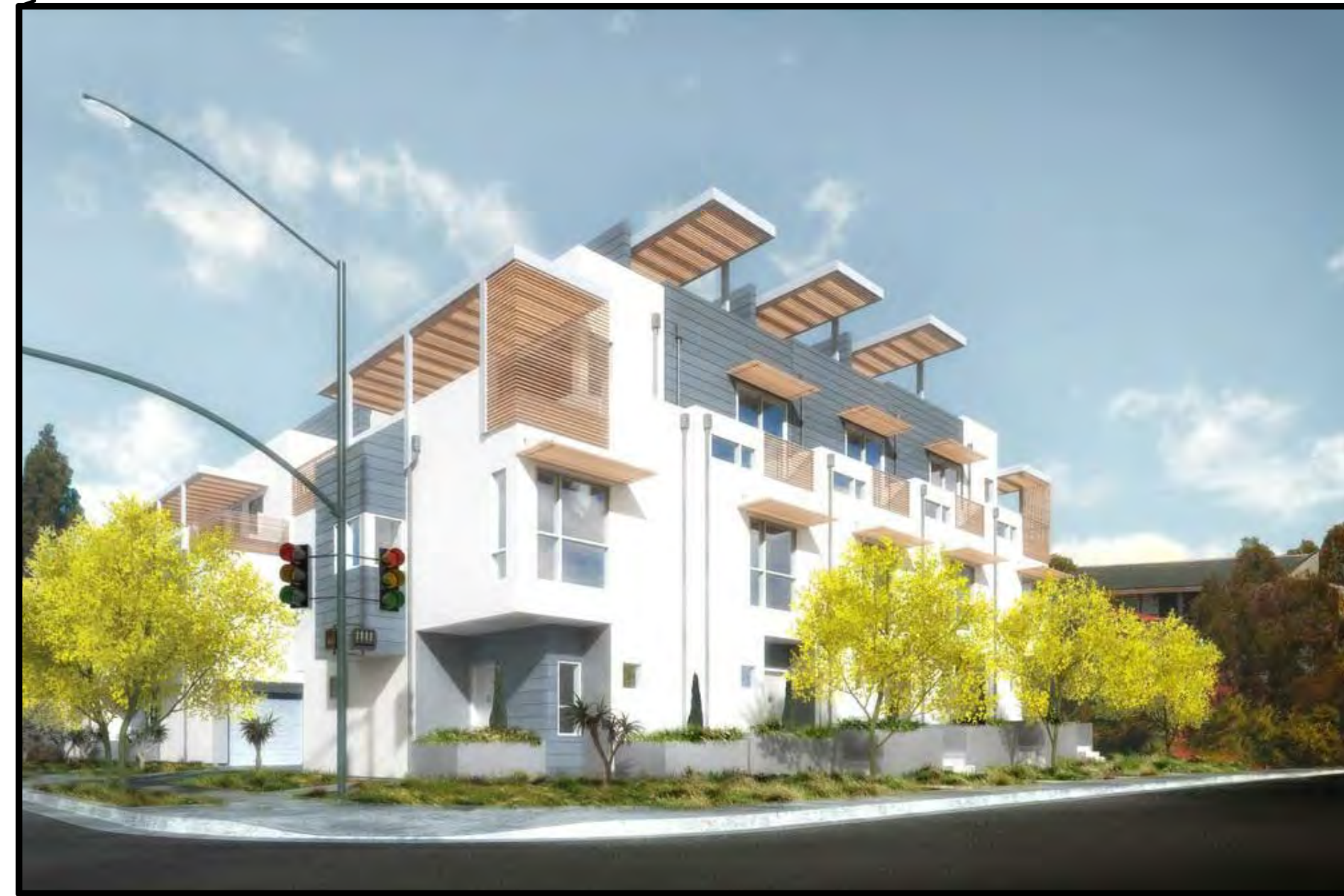
THE GUILD ON 30TH, ON GOING-PROJECT 3 STORY RESIDENTIAL DEVELOPMENT CONTEMPORARY STYLE WITH FLAT ROOF
