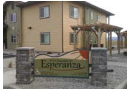
Farmworker housing should provide safe and comfortable living conditions, as shown in this project from Washington State.
