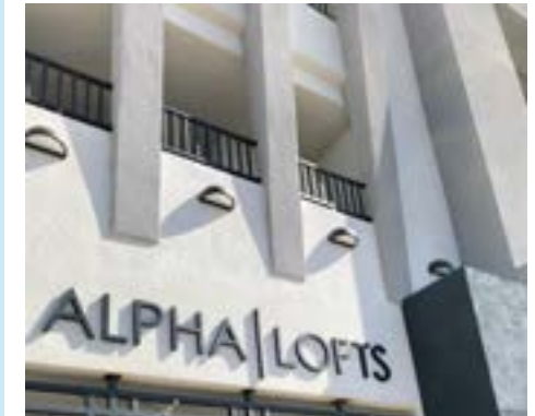
Alpha Lofts is a Veterans Housing development constructed in North Park in 2019.
