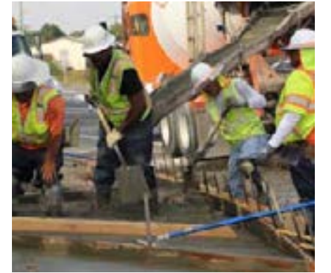
The City can use grants to dedicate funding to priority infrastructure needs, especially in historically underserved communities.
