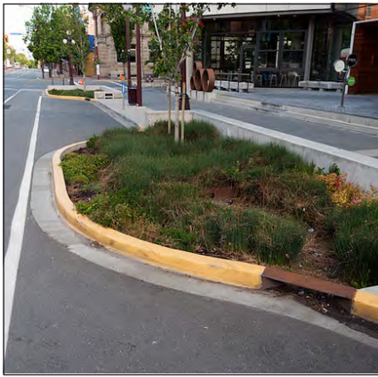
Mid-block Bulbout with Bioretention Soil and Subsurface Drain
