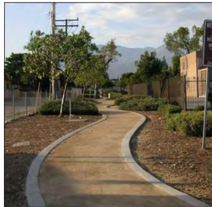
Compacted Decomposed Granite Walkway
