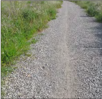
Stabilized Gravel Walkway
