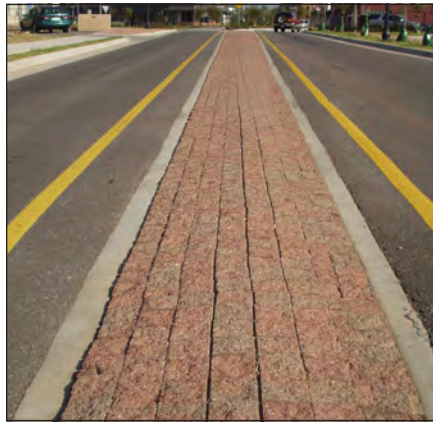
Permeable Paver with Subsurface Filtration and Drains
