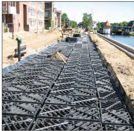
Subsurface Silva Cell and Drain (Use with Permeable Surfaces)
