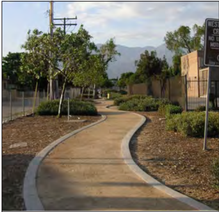
Compacted Decomposed Granite Walkway
