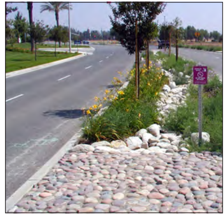
Decomposed Granite/Rock Swale/Gravel Trench
