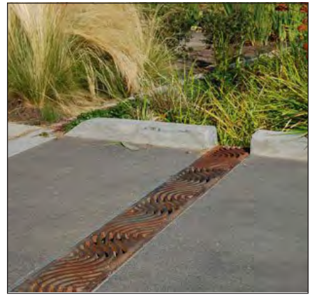
French Drain with Grates
