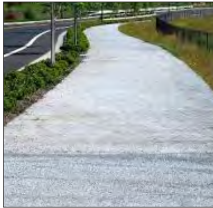
Permeable Asphalt or Concrete
