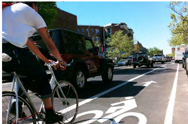
Bike lane next to vehicle lane
