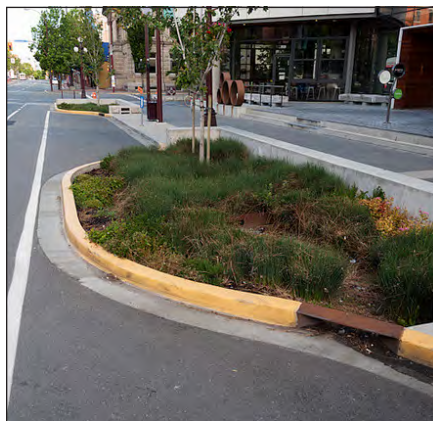
Low Shrubs and Groundcover in a Mid-block Bulbout
