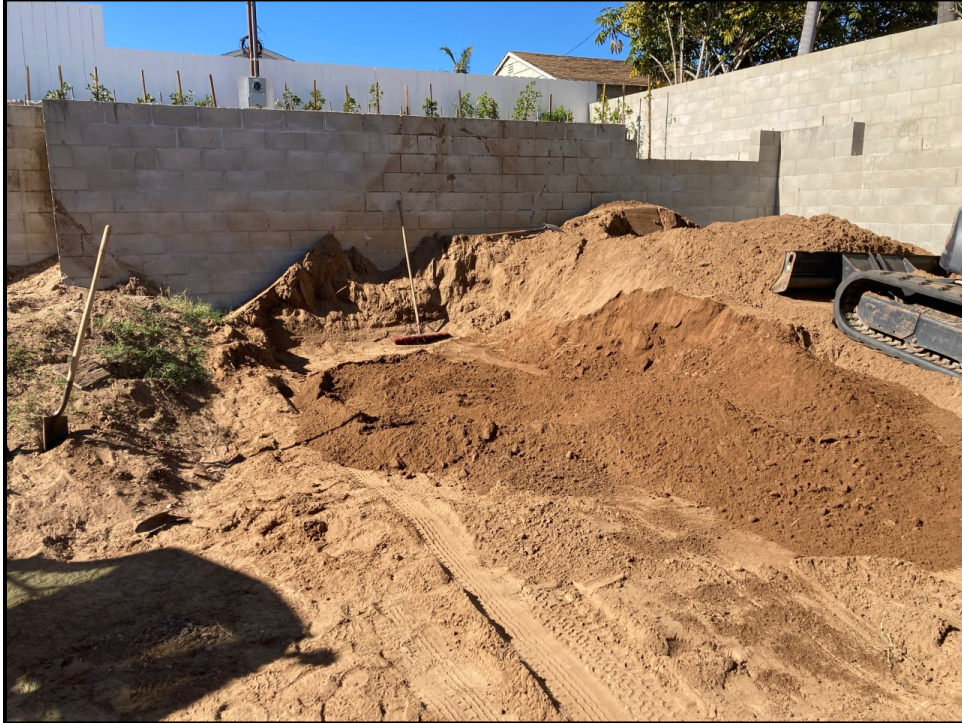
Plate 6.1–1: Stockpiled soil on the subject property for mechanical screening, facing west.
