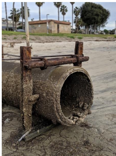
Figure 24. A coastal storm water outfall in San Diego.
