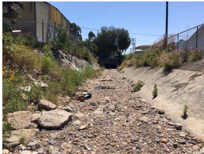
Photo 4. Auburn Channel Maintenance Project (Map 70), post-maintenance, facing southwest, 05/30/2019
