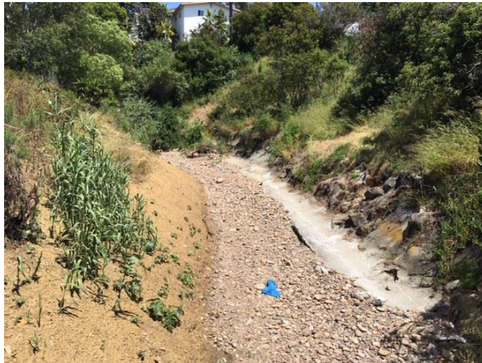
Photo 2. Auburn Channel Maintenance Project (Map 76), post-maintenance, facing east, 05/30/2019
