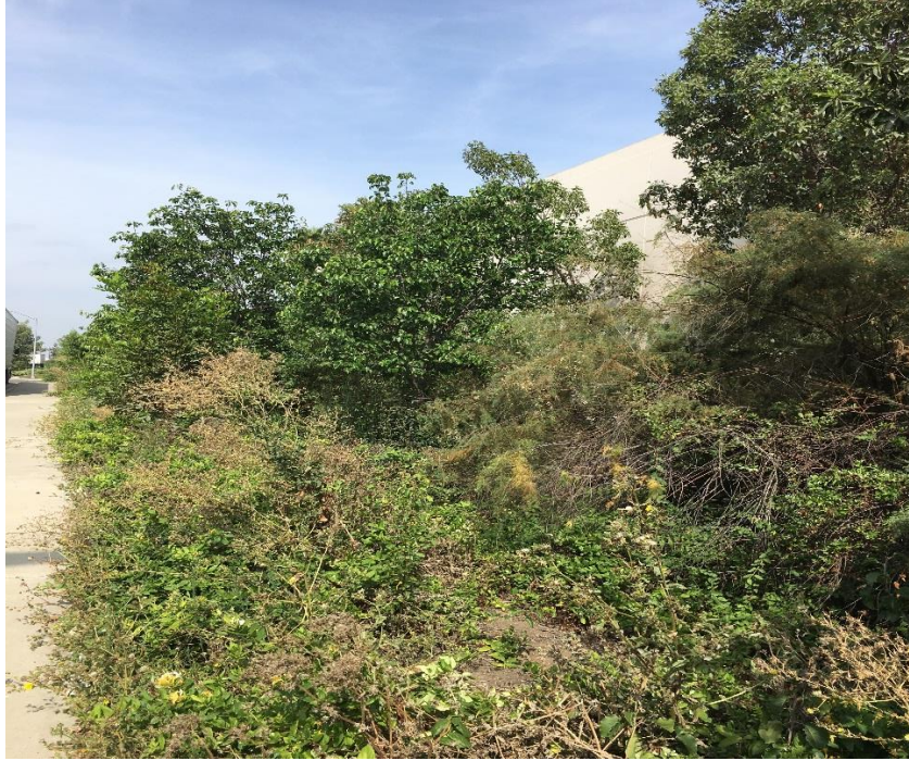
Photo 7. Siempre Viva and Bristow Drainage Facility, pre- maintenance. Facing west from Siempre Viva & Bristow Court cul-de-sac. 8/20/2018.
