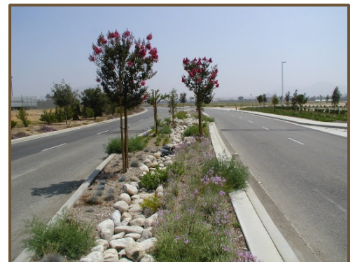
Bioswale within landscaped median.
