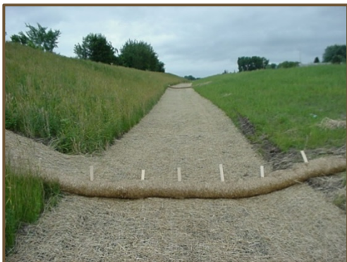
Hay wattles located at 15-foot intervals to stabilize slopes and control erosion.
