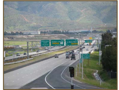
State Route 905 to the north of CENTRAL VILLAGE.
