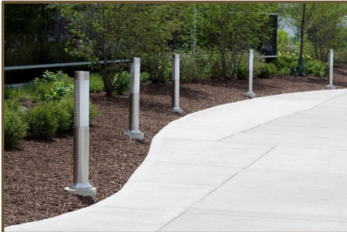
Bollard fixture along pedestrian pathways.
