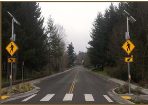
Mid-block crossings provide safe pedestrian crosswalks between intersections.
