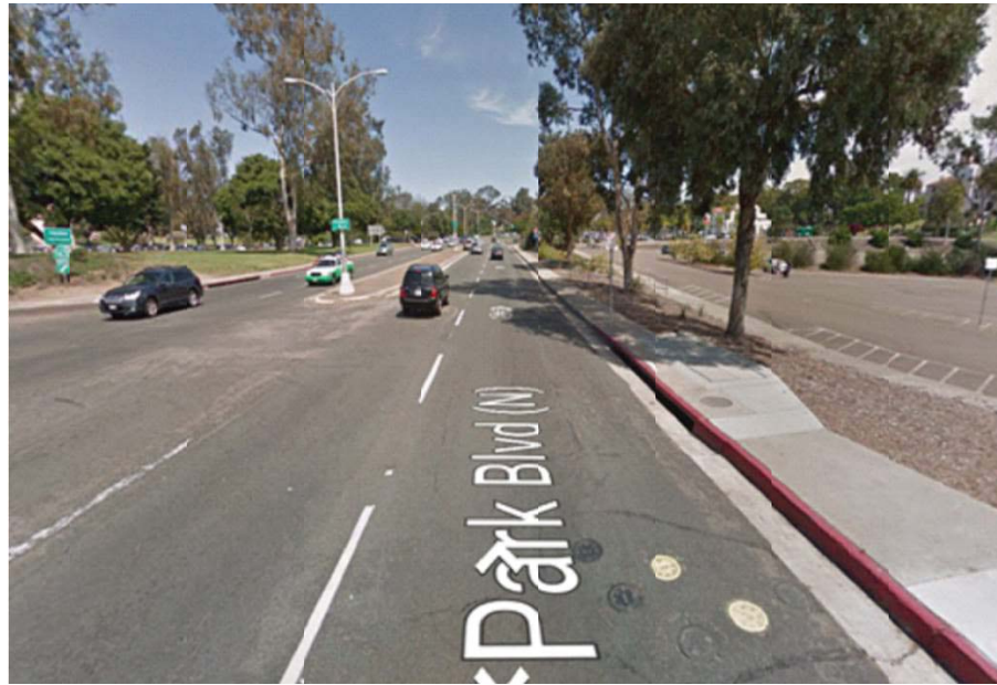
Existing View at Park Boulevard
