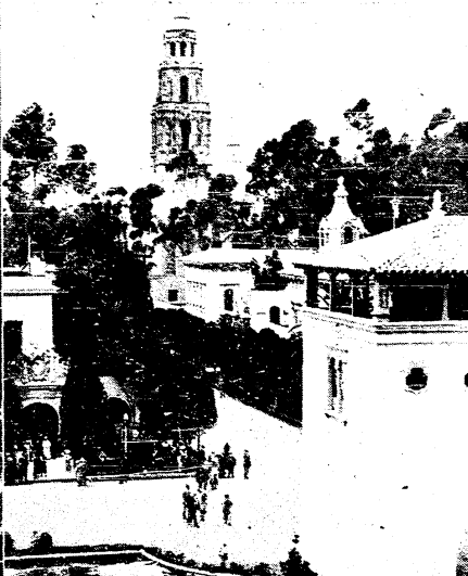
Looking west from the park's central plaza, the California tower is the most striking feature of the landscape. Visible for miles, it is one of the few park buildings thousands of newcomers to San Diego have ever seen. During the war buildings became an annex of the Naval hospital, which with more than 10,000 patients is navy's largest.
