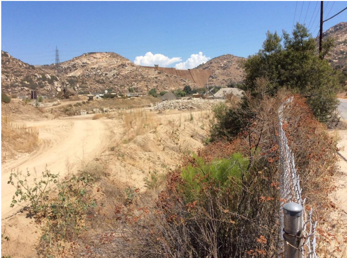
Figure 9. Extensive earthmoving activity within P-37-014654 site boundary, looking northeast.
