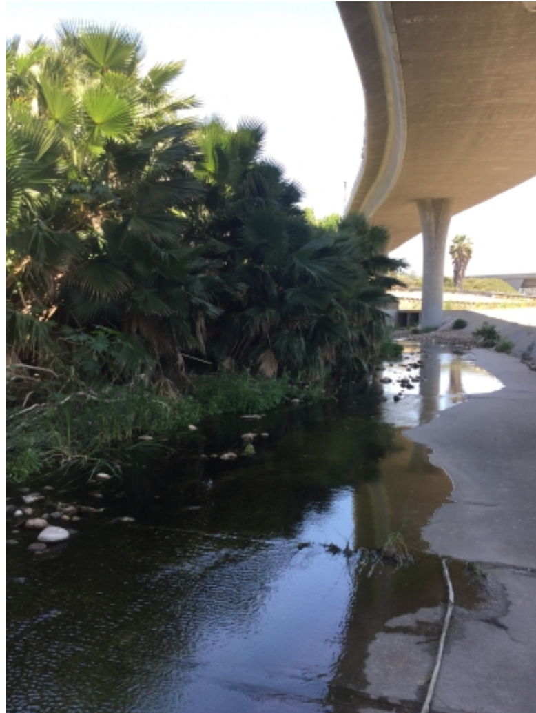
Photo 12: Reach 6 looking upstream (E) under trolley line near Waring Road
