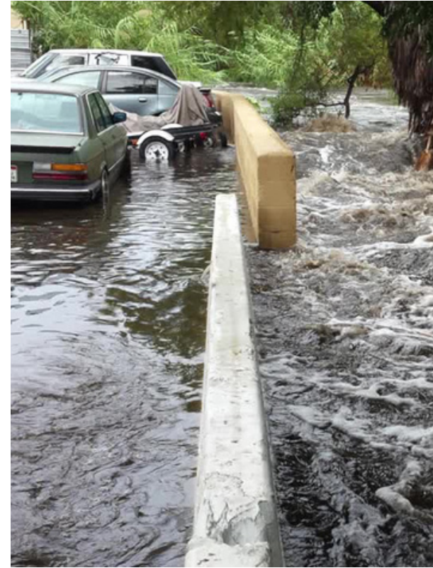
Flooding in the Study Area
