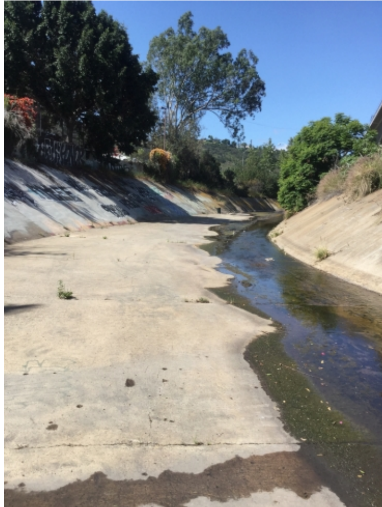
Photo 4: Looking downstream towards Reach 1 (SW) at transition between vegetated and concrete lined channel underneath MTS trolley line
