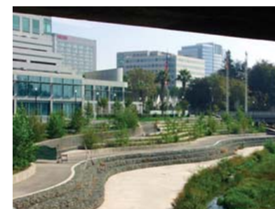
Enhance Channel Sides (gabions)
