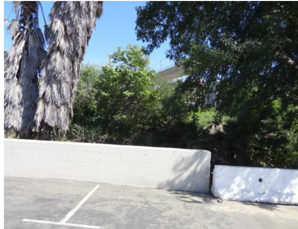
Barricades around Alvarado Creek
