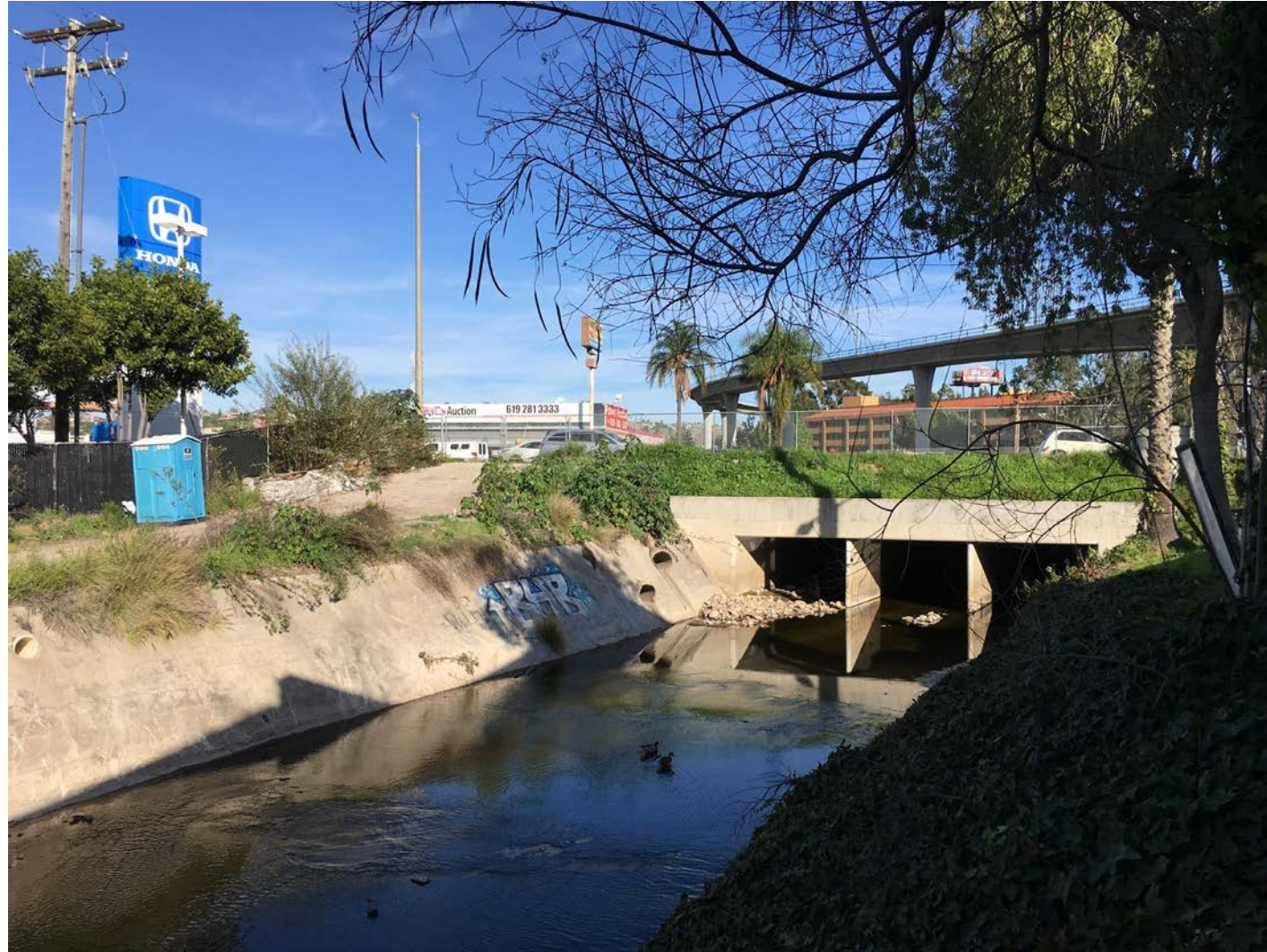
Existing culvert under Mission Gorge Road
