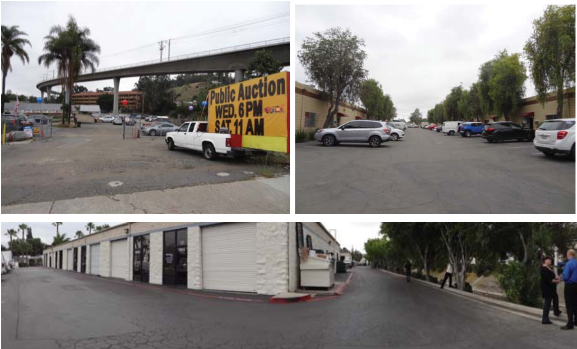
Industrial uses located in the Study Area.
