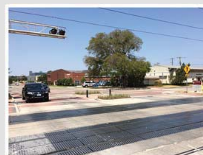
Train crossing is clearly demarcated as a separate area from pedestrian crosswalk
