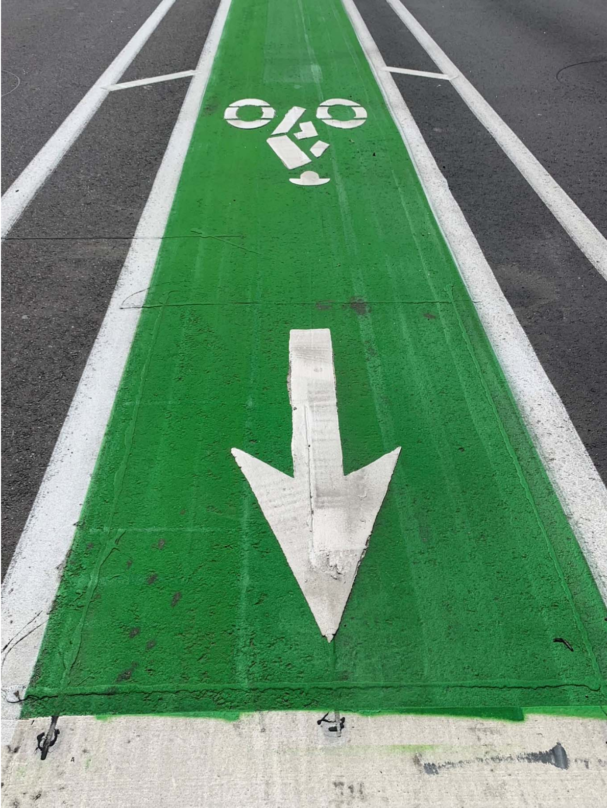
NB Bike Lane on Pacific Hwy just south of Rosecrans Intersection (note painted over sealant outlining square detector loop detector).
