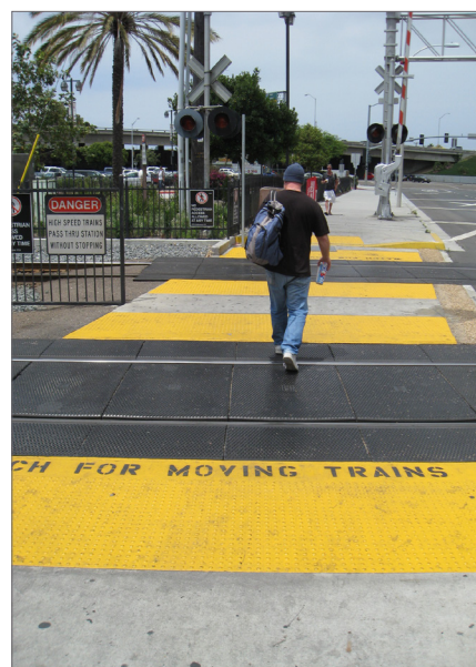
The at-grade rail crossing at the Transit Center on Taylor Street can be improved to reduce crossing delays and enhance safety.
