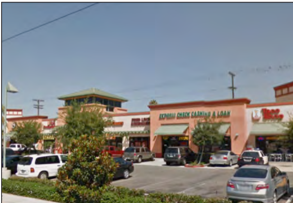
Figure 5.15-8: Strip commercial in Southeastern San Diego
