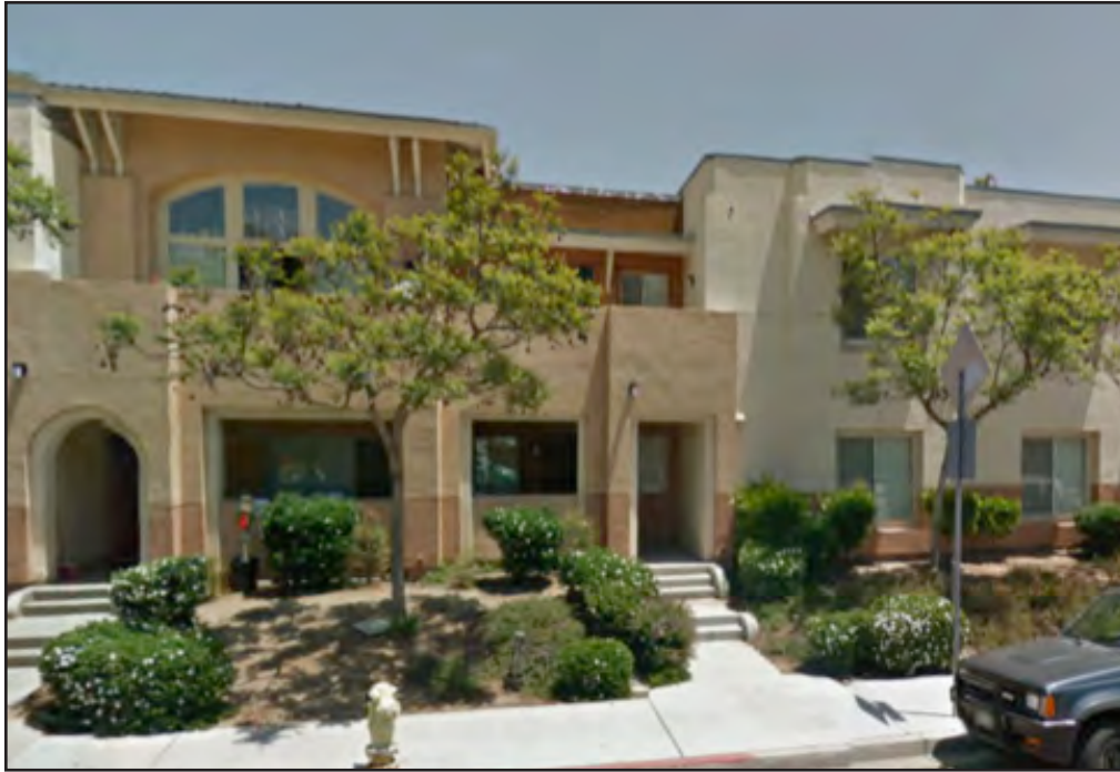
Figure 5.15-7: Multi-family home in Southeastern San Diego
