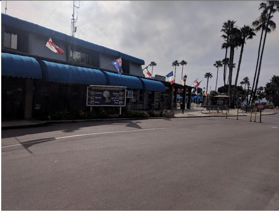
Photograph 7 Campland on the Bay Administration Building, view to northeast, IMG_20180622_090113
