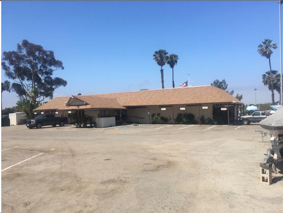
Photograph 10 Mission Bay Boat and Ski Club House, view to southwest, IMG_1287
