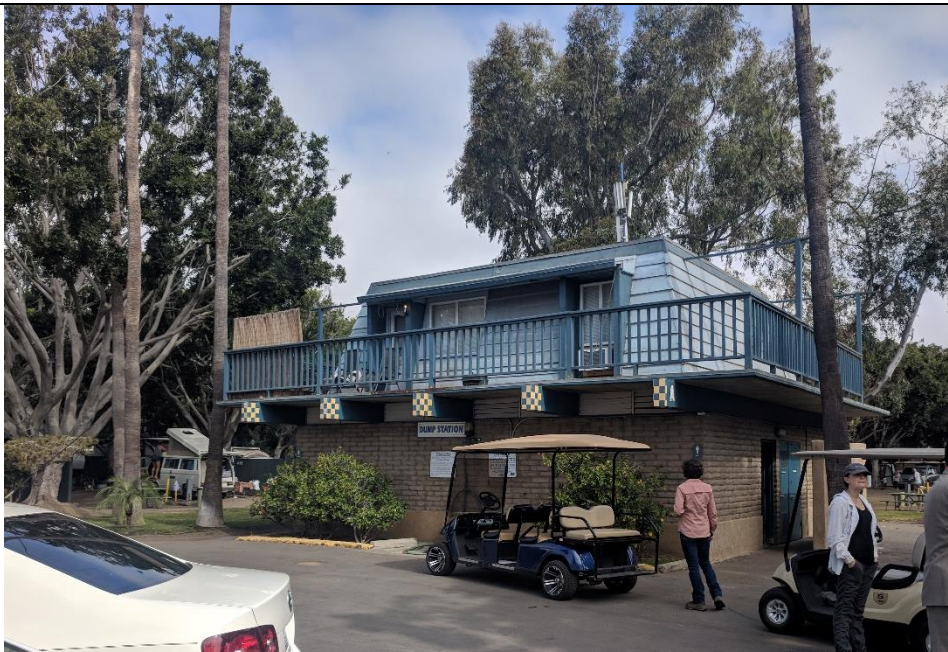
Photograph 8 Campland on the Bay Restroom, view to northwest, IMG_20180622_091442
