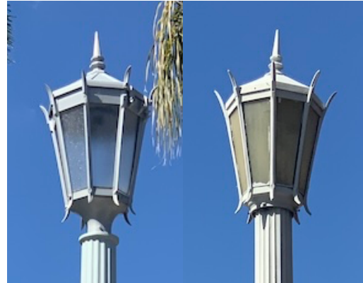
New LED Empire fixture vs yellowed opaque glass of existing light
