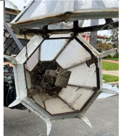
Bulb socket requires replacement. Frame corrosion.
