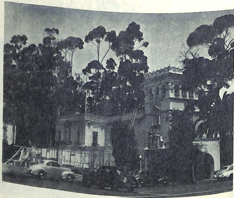
Demolition Of Temporary Structures Erected By The Navy In The Park
