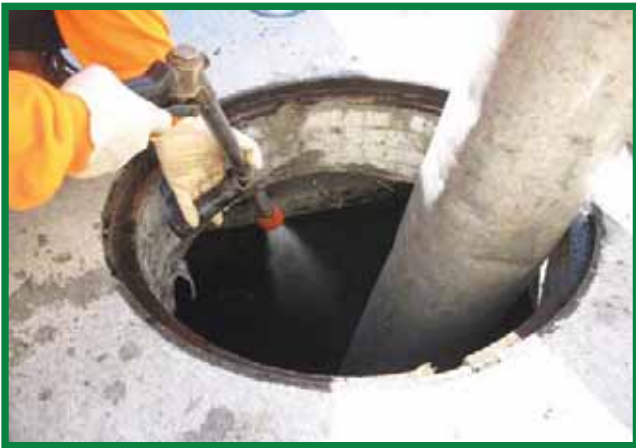
Vacuum out the Sediment Chamber
