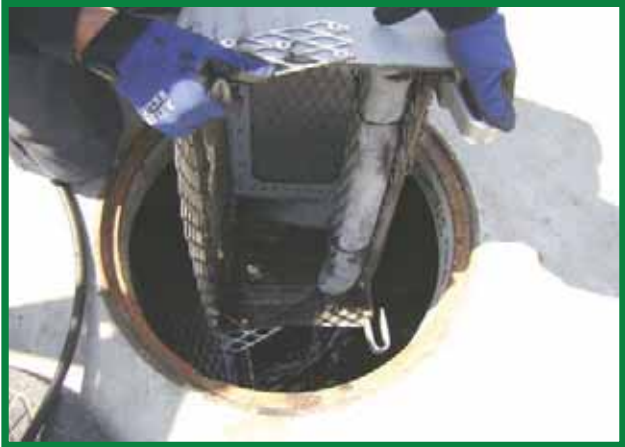
Remove Catch Basin Filter
