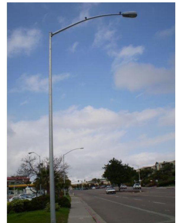
Streetlight & Sidewalk Improvements
