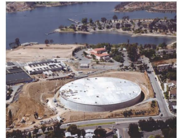
Alvarado Water Treatment Plant
