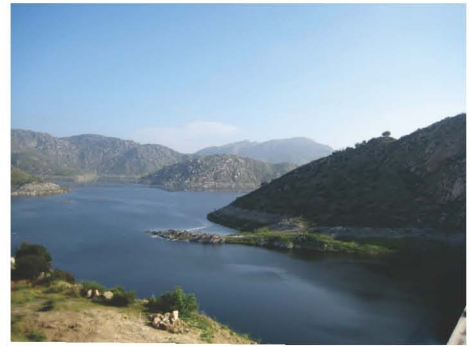
San Vicente, the region's largest reservoir
