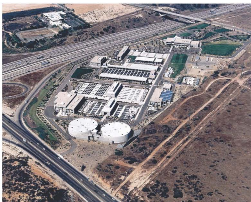
North City Water Reclamation Treatment Plant
