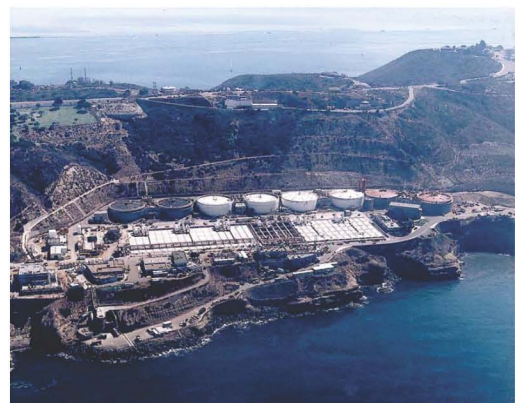
Point Loma Wastewater Treatment Plant
