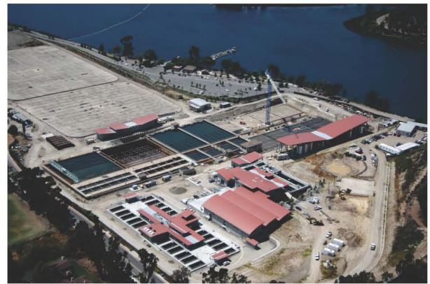
Miramar Water Treatment Plant
