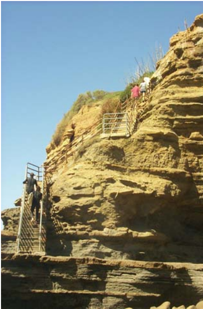
Existing Ladera Street stairs.
