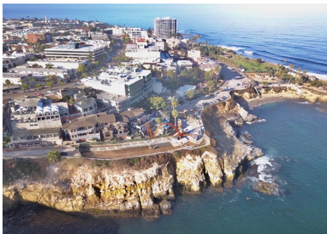
Coast Sea Cave Emergency Stabilization Project
