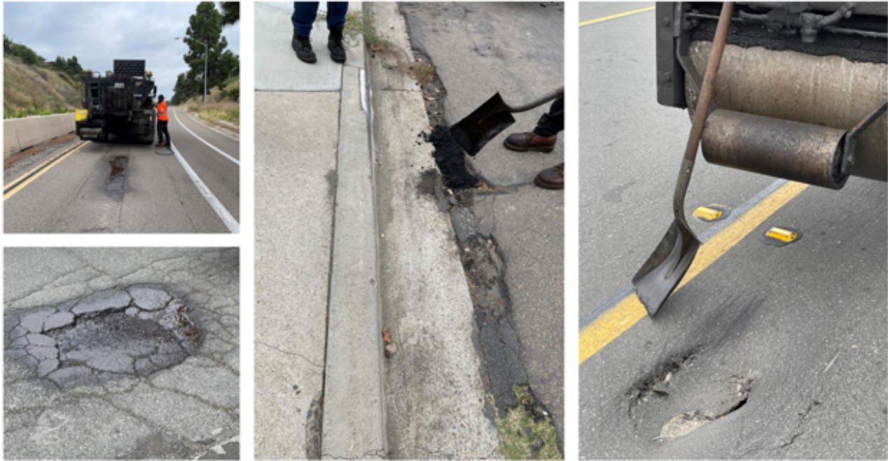
Source: OCA generated from a ride-along with a pothole repair crew.
