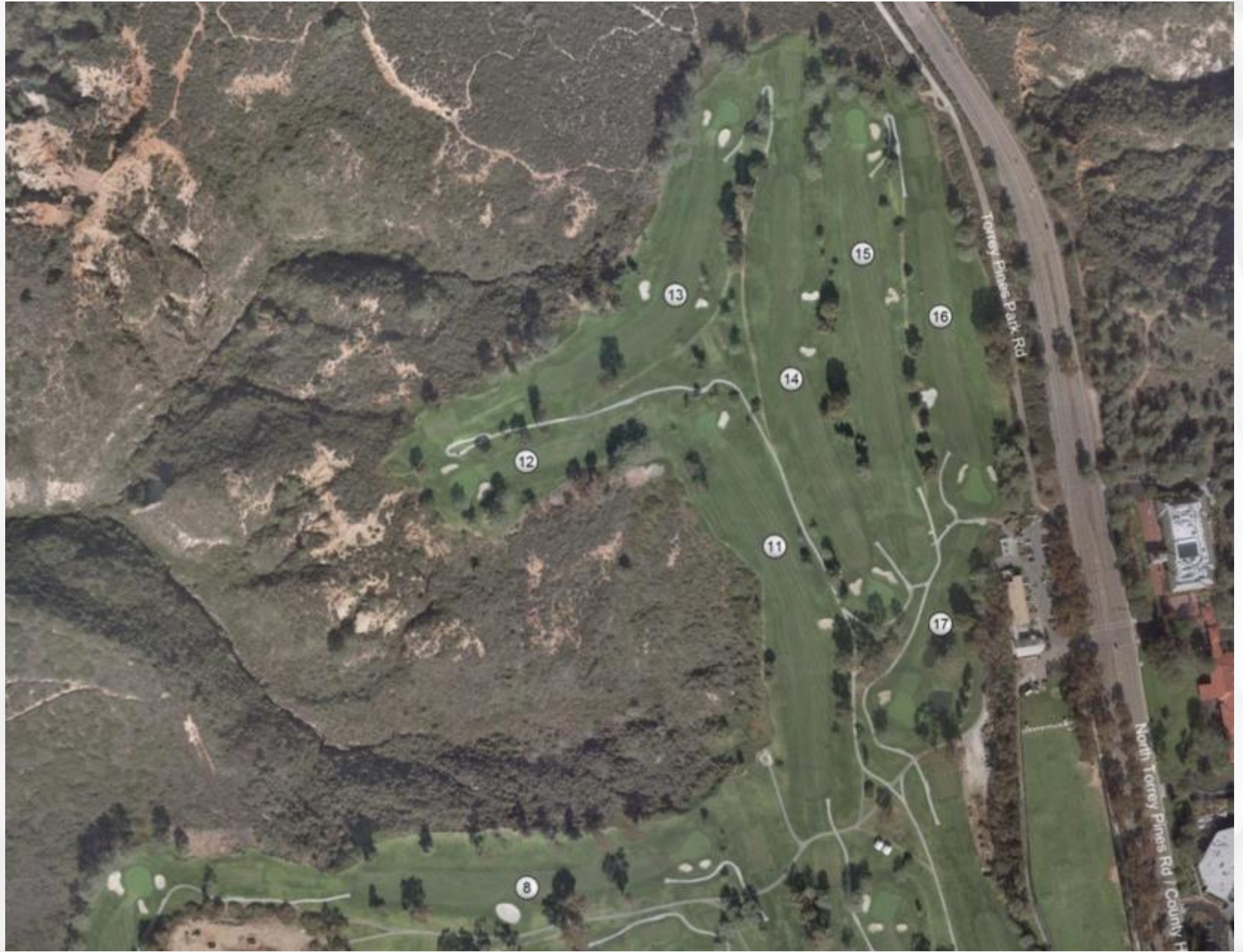
Existing Holes 11 thru 17
