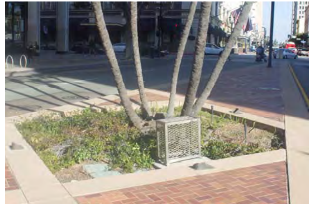
This landscaped median on Broadway is used to catch storm water runoff.
