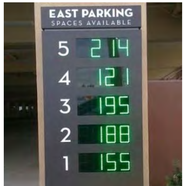
Dynamic signs can be used to display the location and quantity of available parking spaces.
