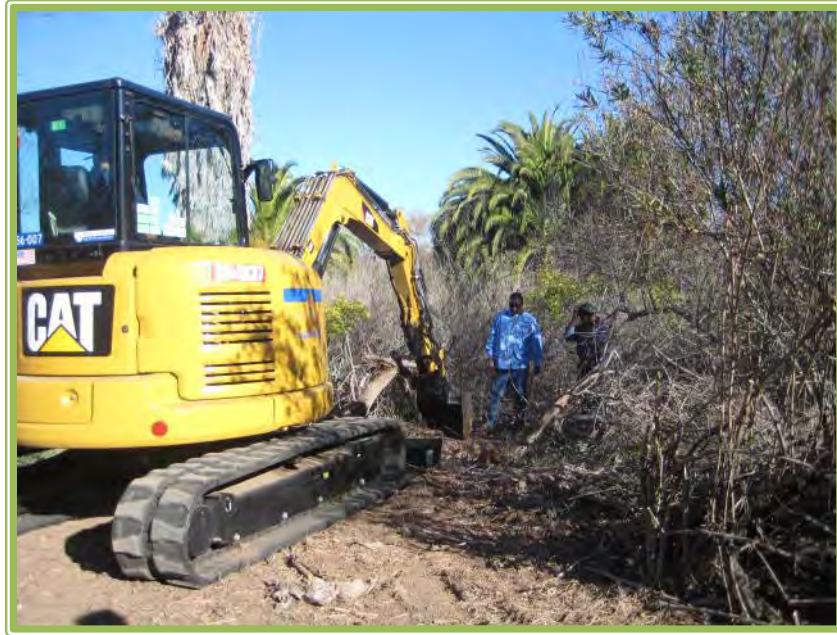
San Diego River West Manhole Raise and Cleaning
