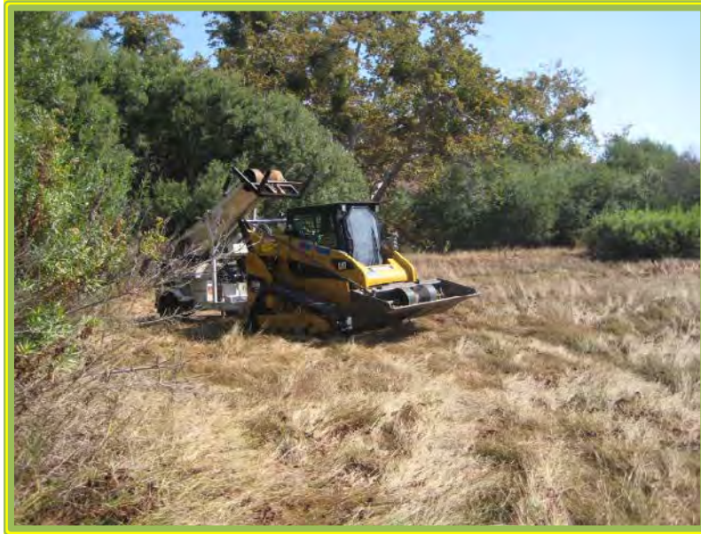
Lopez Canyon –Towing Cleaning Equipment to Manhole 13
