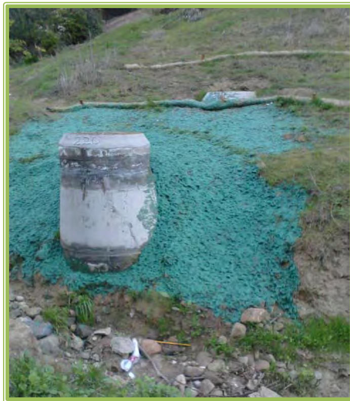
Spruce MH 220 Replacement Revegetation (erosion control) Project
