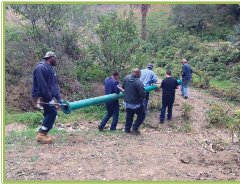
Spruce Canyon Pipe Repair
