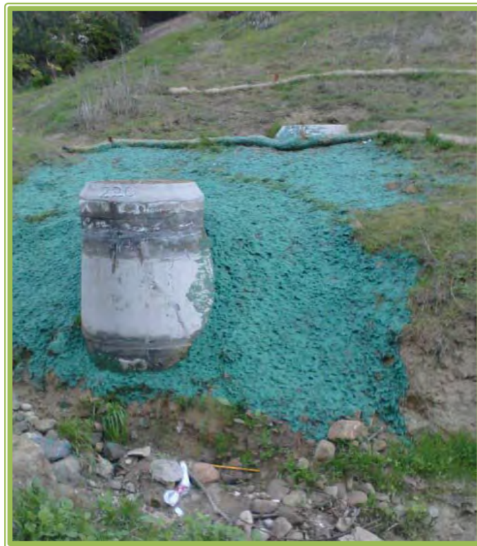
Spruce MH 220 Replacement Revegetation (erosion control) Project
