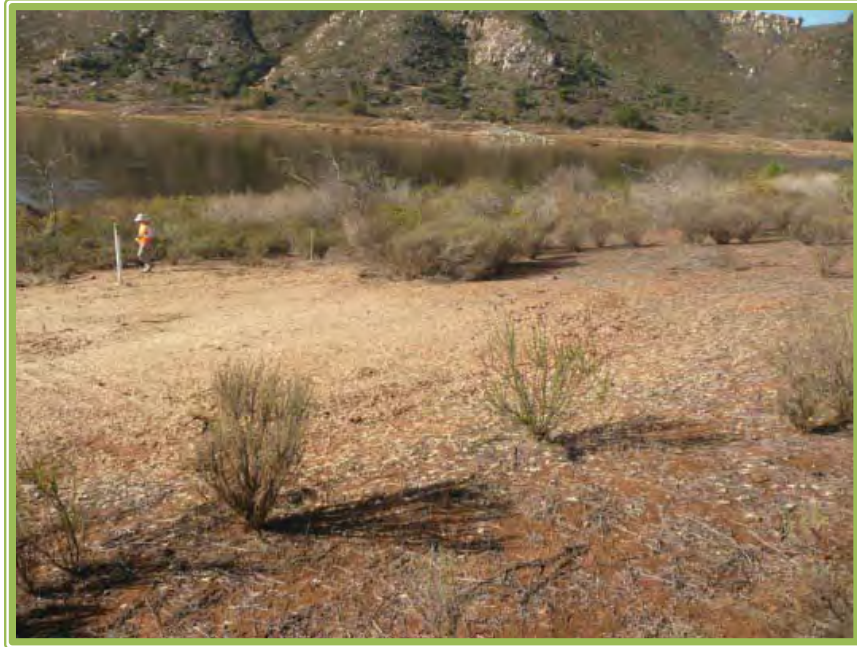
Pump Station 77 Forcemain Restoration Area
