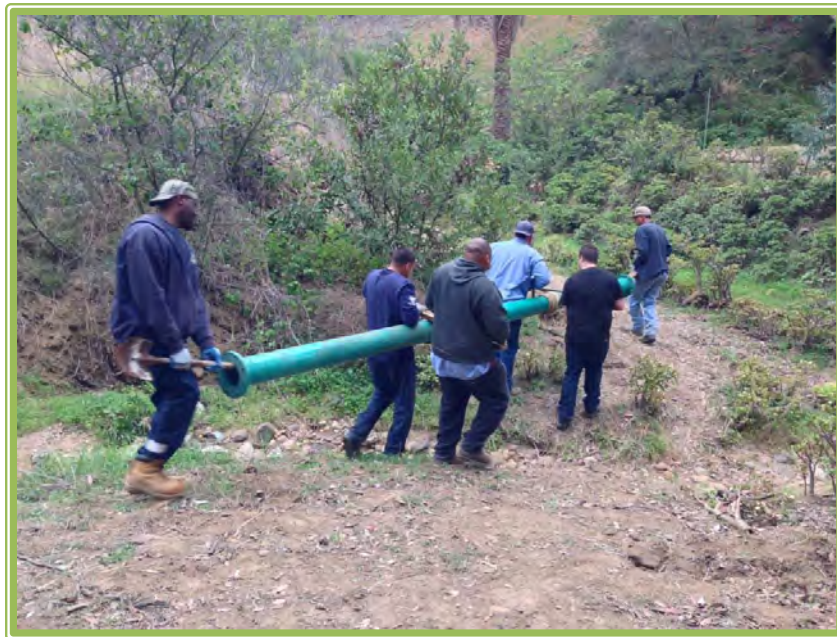
Spruce Canyon Pipe Repair
