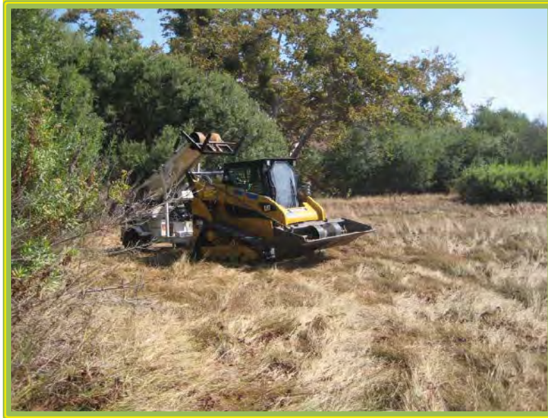
Lopez Canyon –Towing Cleaning Equipment to Manhole 13
