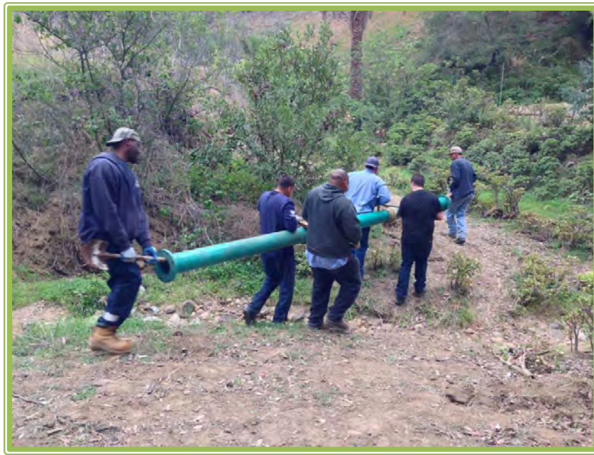
Spruce Canyon Pipe Repair
